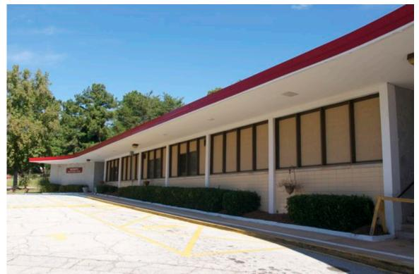
Figure 40: Wadsworth Elementary's front windows have been replaced and covered over
