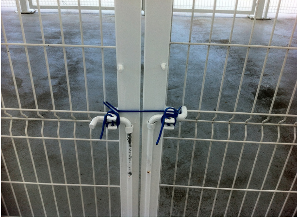
Gates must be opened and manned once spectators are inside the stadium. Failure to open gates during mass evacuation leads to loss of life.
