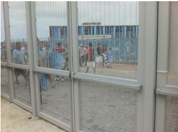
Gates that open easily from the inside, yet adequately prevent entrance from the outside are the safest form of exit.
