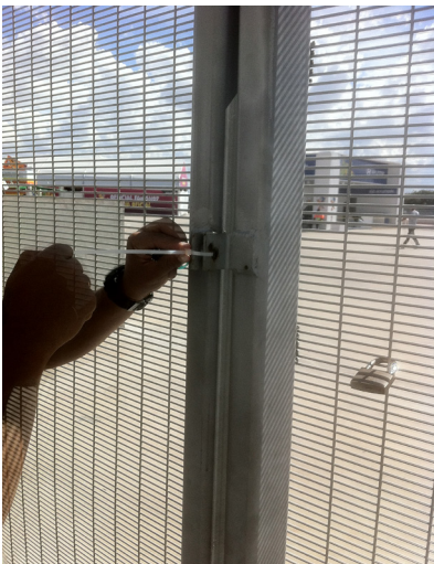
It is preferable to unlock all exits and replace the lock with cable ties, as these can easily be overcome by a crowd wishing to exit in an emergency.
