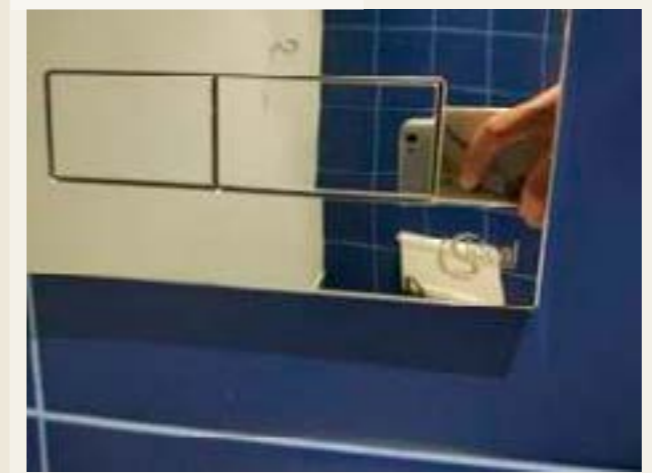
Fig. 29. Water-saving sanitary fixtures in Nizhny Novgorod Stadium
