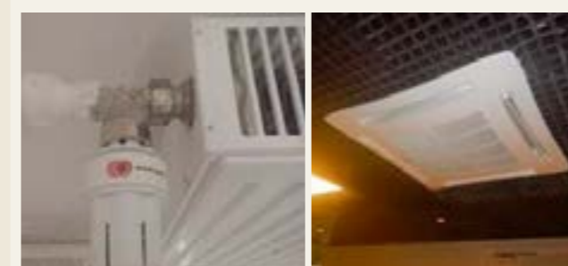
Fig. 10. Thermostatic valve and fan-coil unit in Luzhniki Stadium
