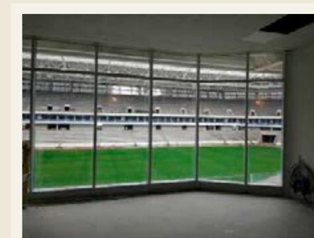
Fig. 3. Glass structures of Kaliningrad Stadium
