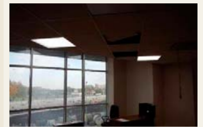
Fig. 36. Glass structures of the Mordovia Arena
