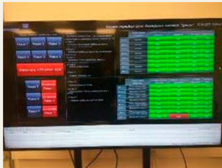
Fig. 14. Lighting control in Luzhniki Stadium on the dispatcher panel
