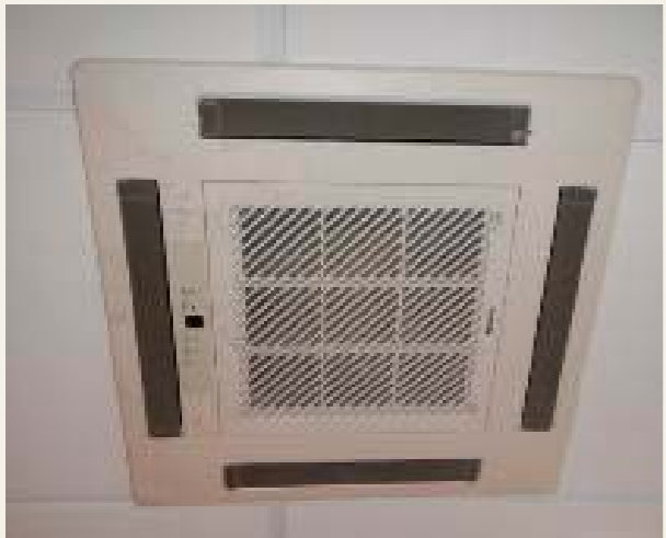
Fig.37. (1) Radiator (thermostatic valves are being installed). (2) The installed fan-coil unit
