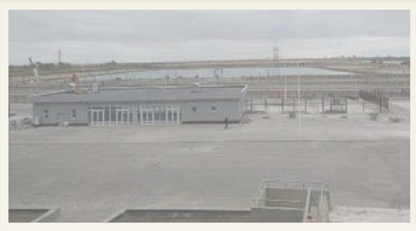
Fig. 24. Rainwater collection tank
