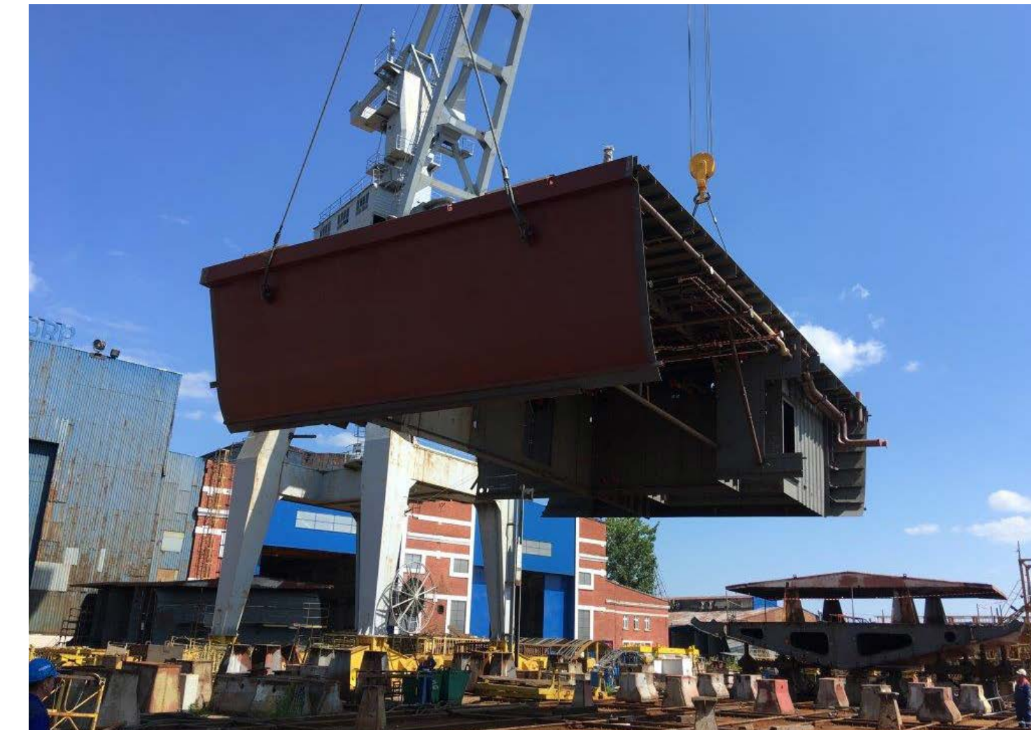
Craning a section of hull into place
