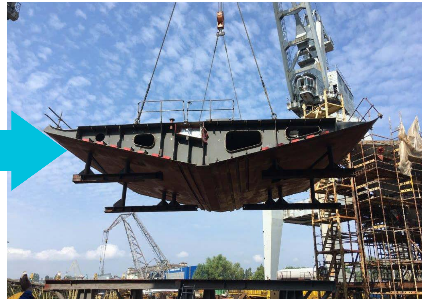
A section of the keel is dropped in place
