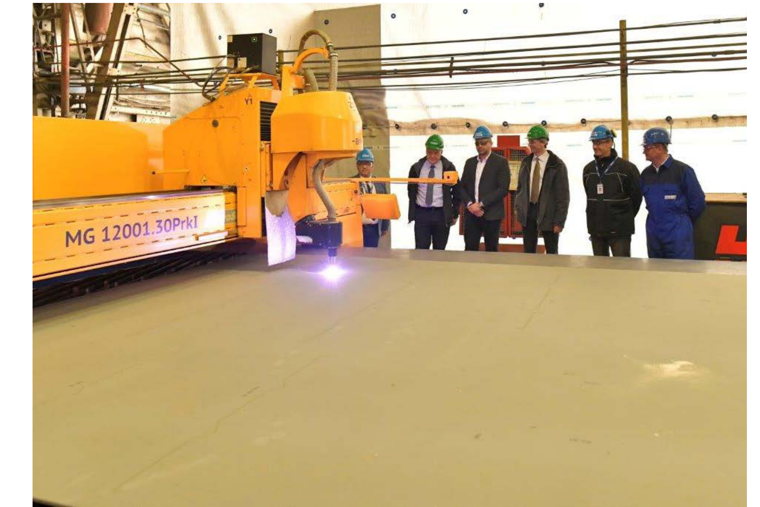
The build begins!
