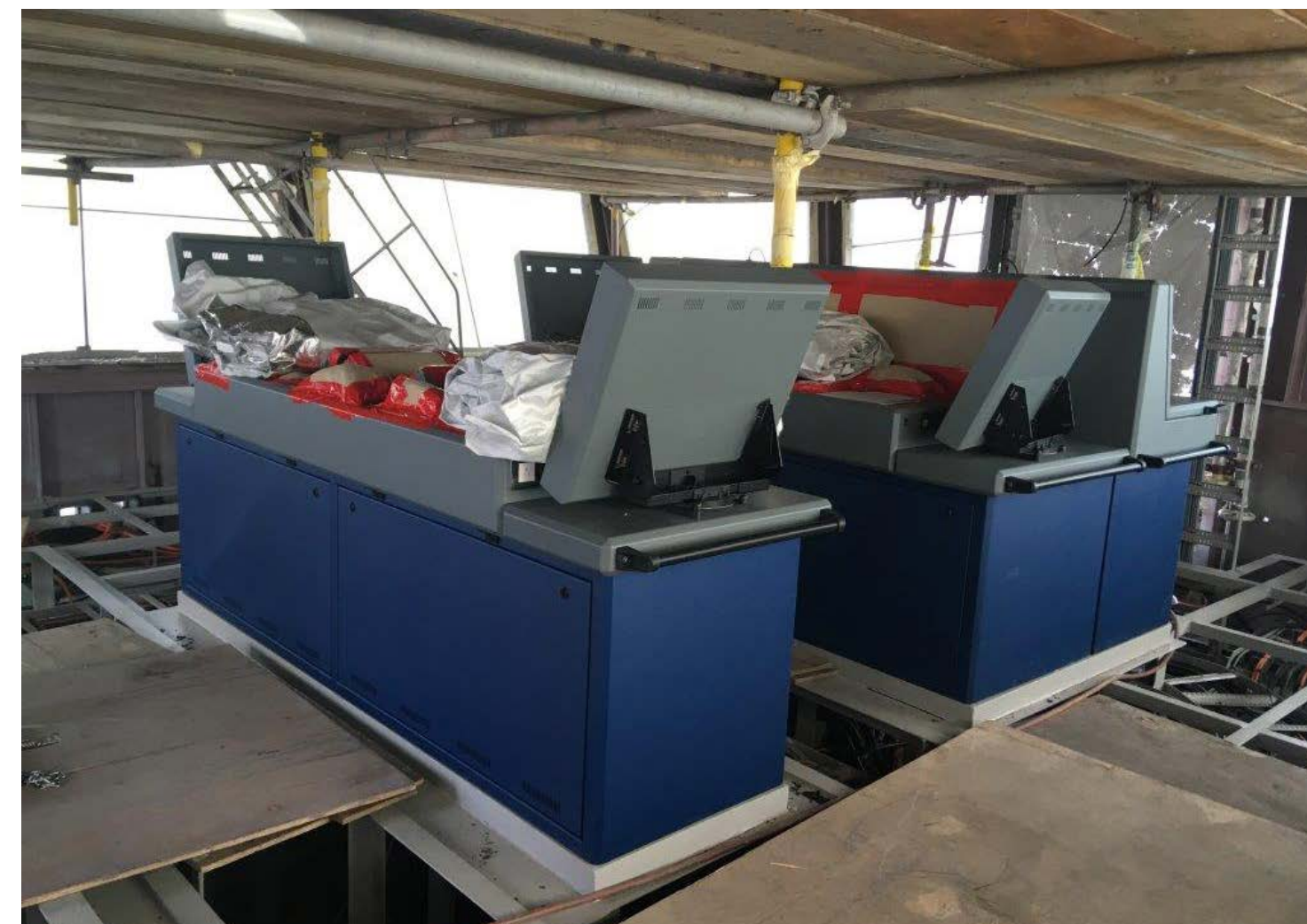
Installing the navigation equipment
