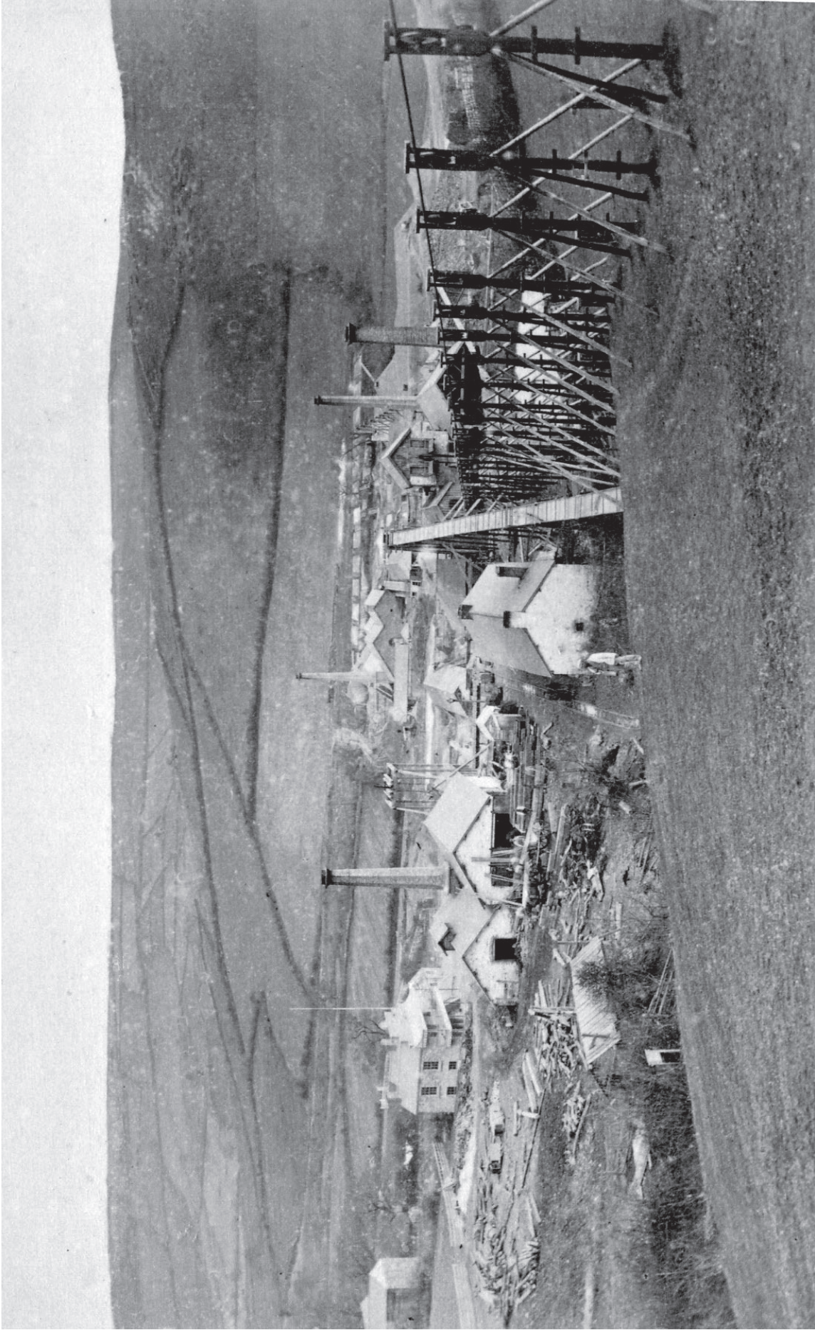
Figure 3. ca. 1870. This superb photograph was taken looking down the hillside to the south. It shows the newly constructed buildings of the mine with the offices to the left. On the right is the flat rod system from the Mary Emma waterwheel to the Engine Shaft which operated the pumping and winding plant of the mine. This system was replaced in 1876 when the Cornish pumping engine was built and, therefore, dates the photograph prior to that date.
