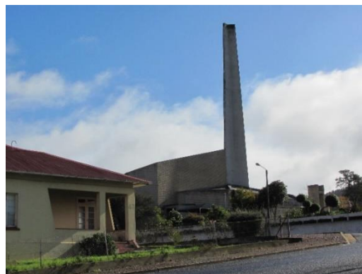
Figure 53: Street view of Caledon West Dutch Reformed Church, Conradie, 1978 in 2015. Photograph by the author.
