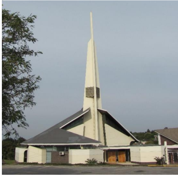
Figure 37: Exterior of the Uitenhage Winterhoek Dutch Reformed Church, A.P.S. Conradie, 1977 in 2015. Photograph by the author.
