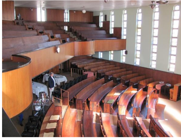
Figure 13: Interior of Bellville Dutch Reformed Church, J.Anthonie Smith, 1940 in 2016. Photograph by the author.
