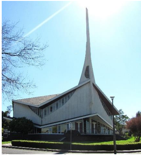
Figure 31: Exterior of Parow Oostersee Dutch Reformed Church, A.P.S. Conradie, 1973 in 2015. Photograph by the author.
