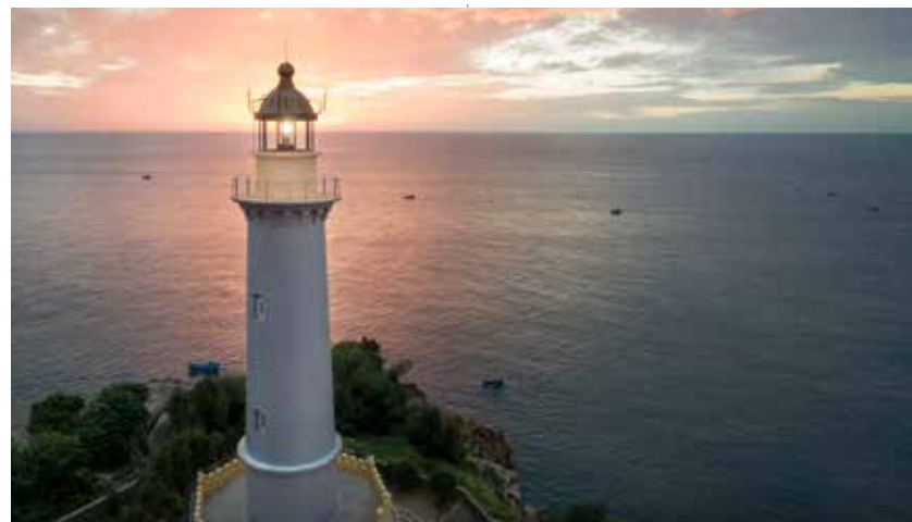
During 2018, our Dulux Weathershield paint was applied to Vietnam's Dai Lahn lighthouse, which is more than 100 years old. The tough, ultra-protective coating will help the historic structure to cope with anything the elements decide to throw at it.
