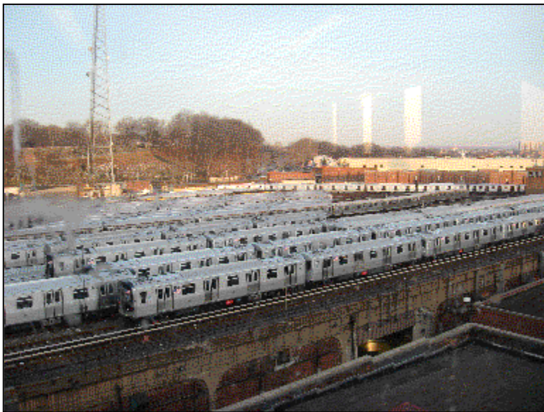
East New York Yard from the L Line overpass to the Manhattan-bound platform. Graffiti mars the left edge of the photo.
