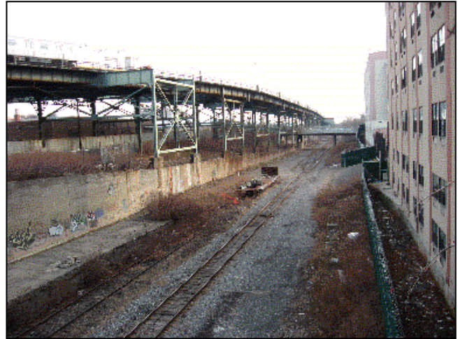
Rebuilt by two separate corporations in the early 20 th century, today's L Line viaduct (left) and the NY&A Bay Ridge freight line (right) operate redundant rights-of-way which can be consolidated, reducing maintenance costs and opening up more space for potential reuse.
