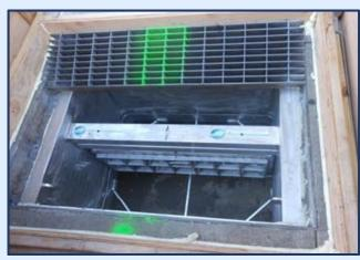
Mechanical Closure Device Vent Cover
