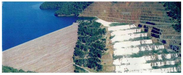
Figure 5 Dartmouth Dam during spilling down the quarry benches
