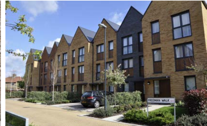
Allocated forecourt parking at Kidbrooke screened by well maintained planting
