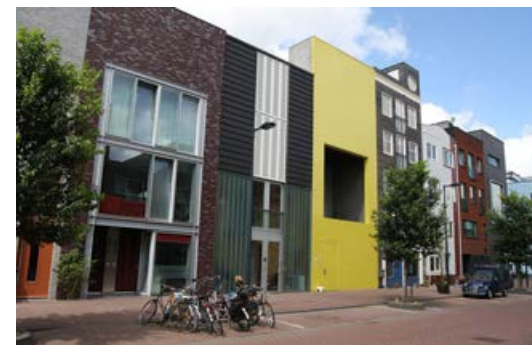
Example for custom build housing - Ijburg, Amsterdam (photo by Peter Visser)
