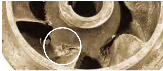
Cavitation corrosion of bronze impeller
