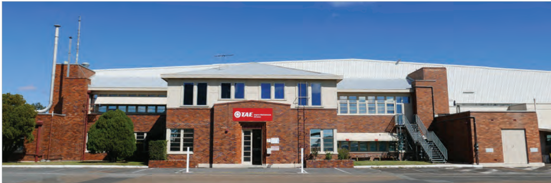
Hangar 76, constructed at RAAF Base Amberley in 1939. (RPS 2015).
