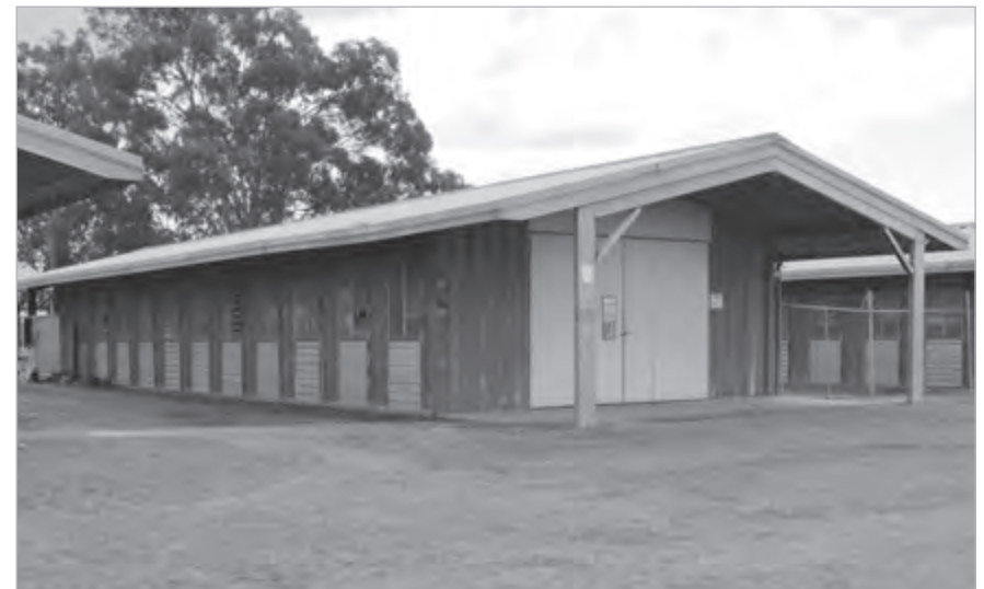
A Lysaght hut, one of a group of ten, known as 'Silver City', constructed for the 16ALA. (RPS 2016).
