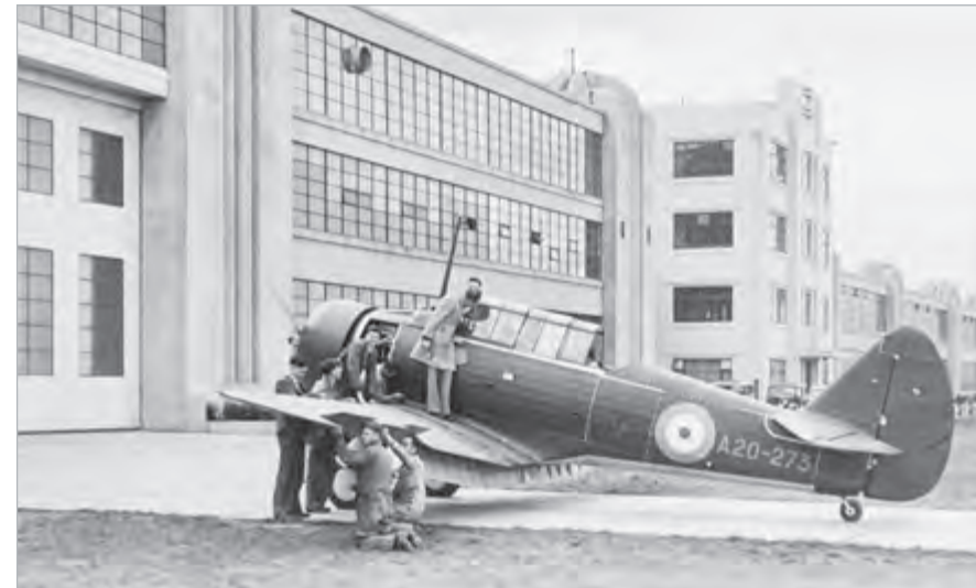
Commonwealth Aircraft Factory, Fishermans Bend, Victoria with Wirraway nearing completion, c.1941.
