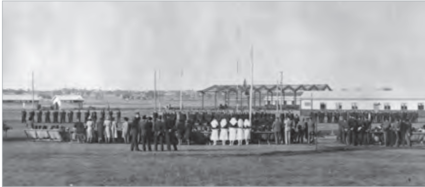
Amberley Parade 1940s with Hangar 76 under construction in the background. (23SQN Historian).
