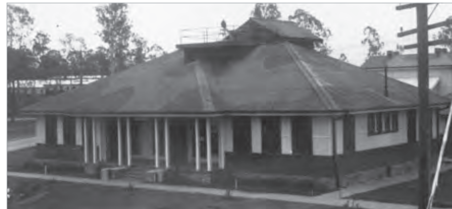
Station Headquarters in 1940s with roof painted in camouflage colours. (RAAF Museum, Point Cook).
