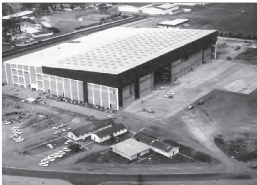
Building No 363, known as the Taj Mahal, constructed for the F-111. (RAAF Museum, Point Cook).
