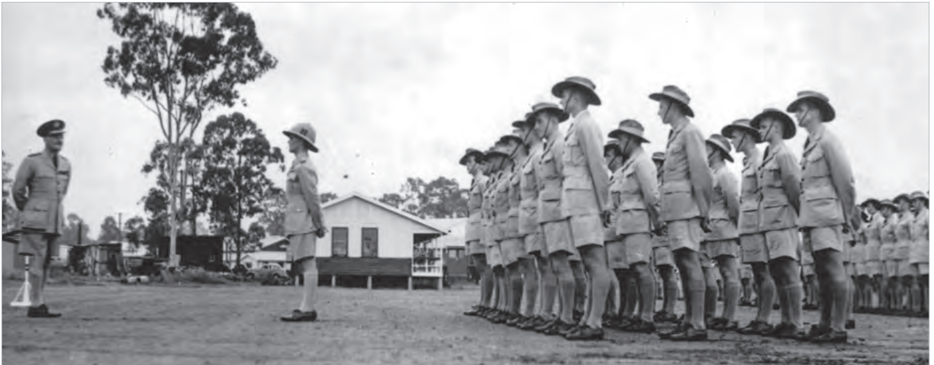
RAAF Base Amberley Parade Ground with hospital ward visible in the background. (23SQN Historian).
