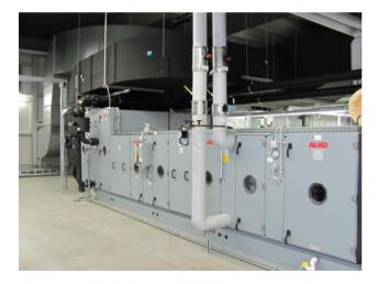
Figure 9: Tunnel Air Handling Unit.
