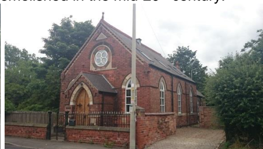
Figure 2.7: Former Wesleyan Methodist Chapel, built 1897.
