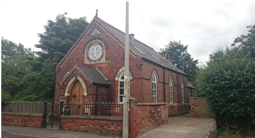
Figure 3.17: Former Wesleyan Methodist Chapel, Top Street, after conversion to a dwelling.
