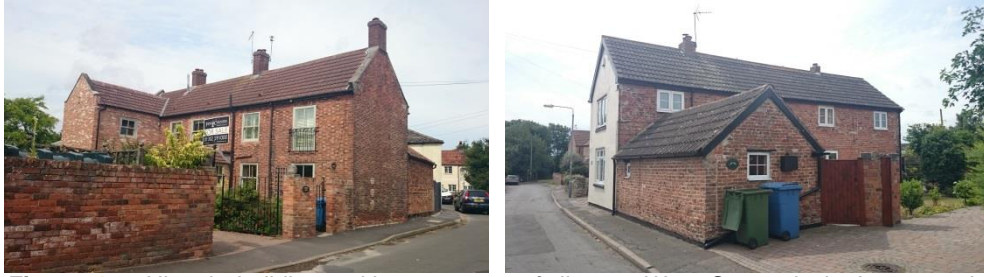
Figure 4.6: Historic buildings with concrete roof tiles on West Street. In both cases, the significance of the building has been harmed by the use of such materials.
