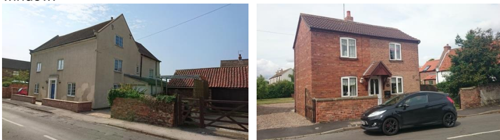
Figure 4.8: The use of standard PVC windows on the building on Middle Street (left) has resulted in the Georgian character of the building being harmed, this harm being added to by the modern render and concrete roof tiles. The PVC windows on the property on West Street (right) fail to reflect the early-19 th century architecture of the cottage and detract from its significance.
