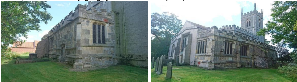
Figure 3.7: Views of north aisle from north west (left) and north east (right).
