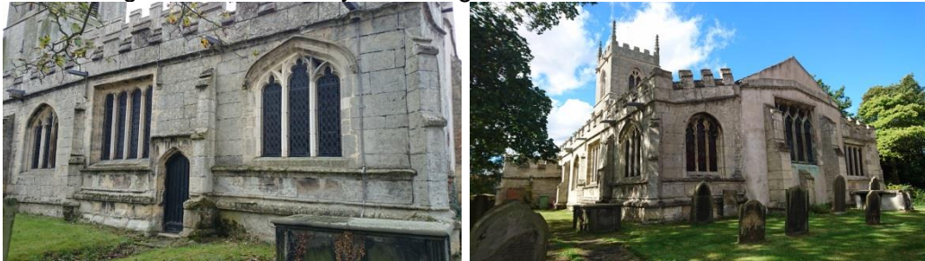
Figure 3.5: Views of south aisle, including Tudor square-headed window opening (left).
