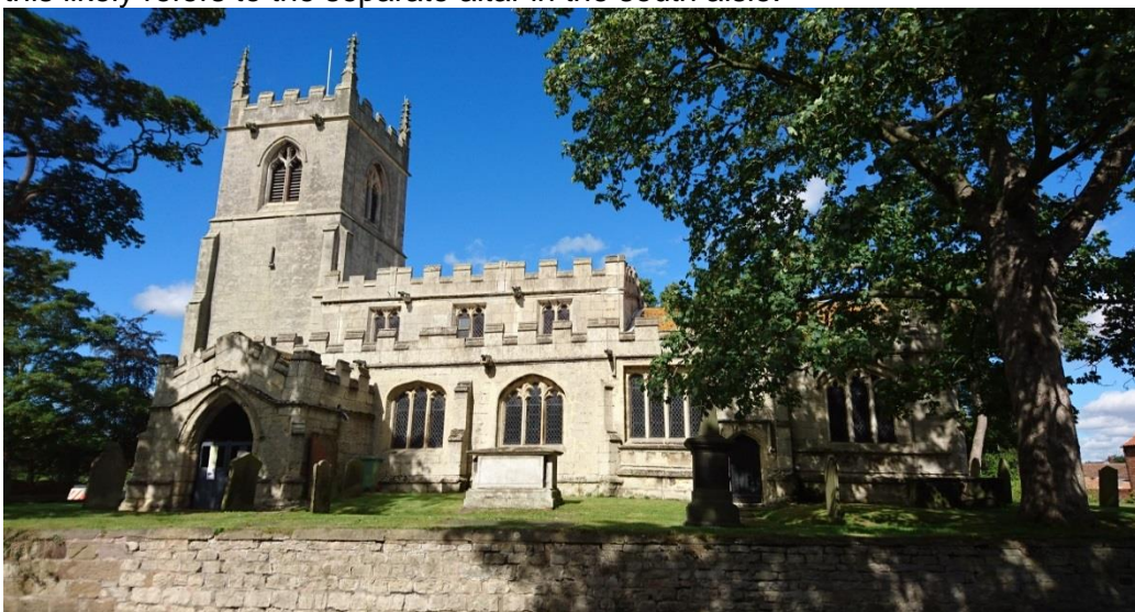
Figure 2.4: St John the Baptist's Church, Misson.
