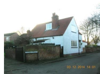
Figure 3.20: The Lodge, Church Street.
