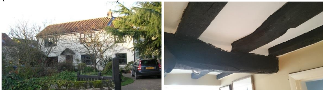
Figure 3.11: Views of façade and internal timber frame at Gibdyke House.
