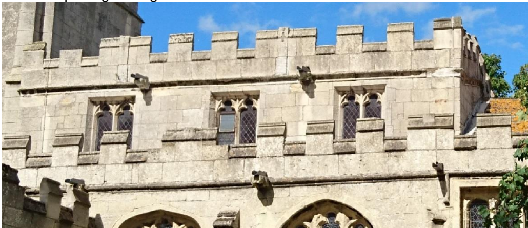
Figure 3.6: Clerestory openings, south side.
