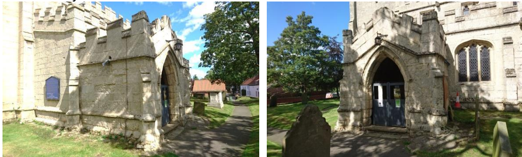
Figure 3.4: Church of St John the Baptist, south porch.
