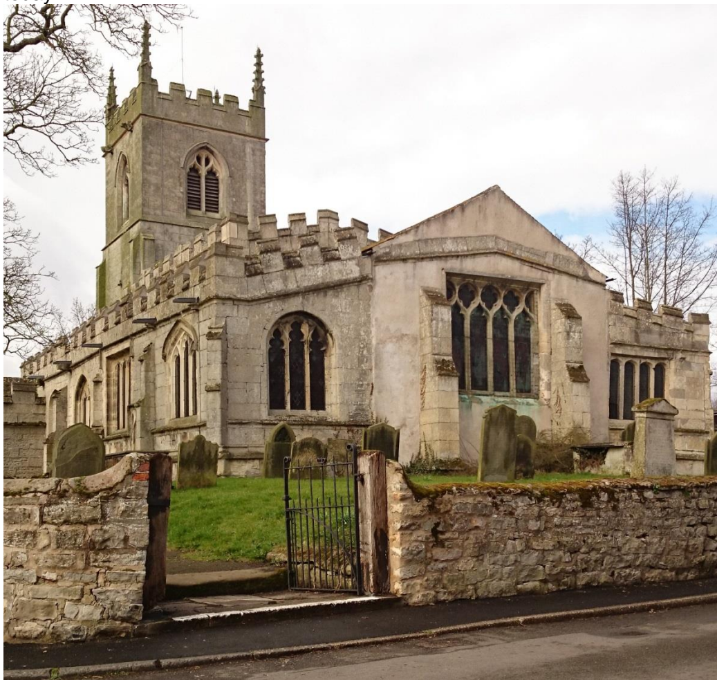
Figure 3.1: Church of St John the Baptist, viewed from south east.
