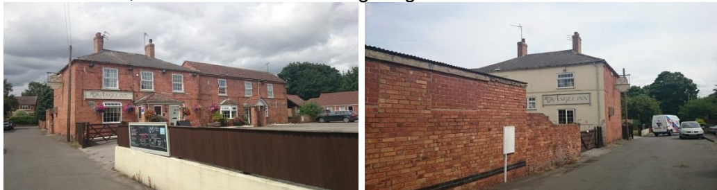
Figure 3.19: Views of Angel Inn, Dame Lane.
