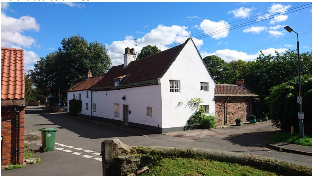
Figure 3.9: White Cottage, High Street (as viewed from churchyard to north west).
