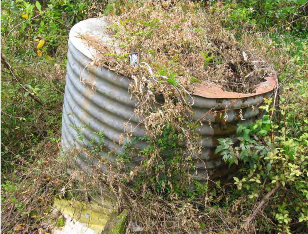
Figure 43 Remains of water tank, WP 125
