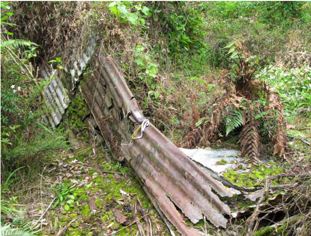
Figure 42 Remains of roof of dwelling, WP 125
