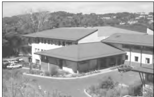
▲ The new building housing the Compton Herbarium.
