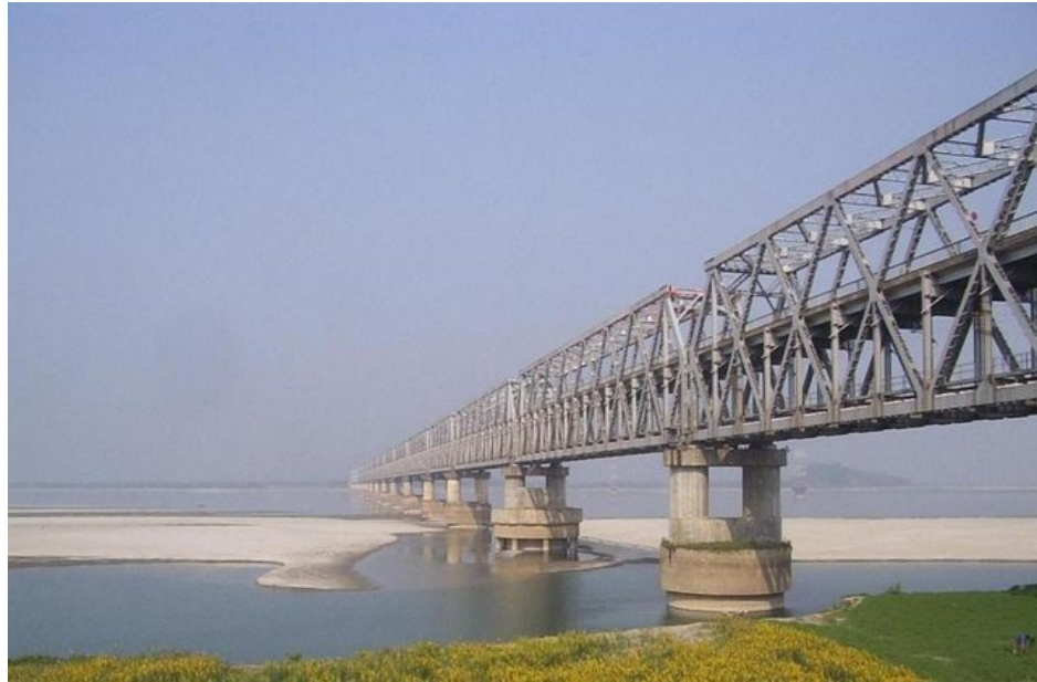
Naranarayan Setu-view of completed bridge
