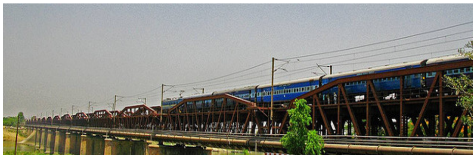
Yamuna Bridge, Allahabad (at present)
