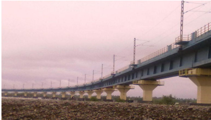
View of completed bridge
