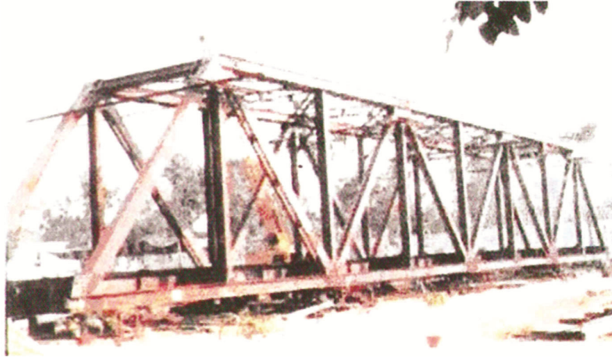
Prototype Erection of 150 Feet Girder
