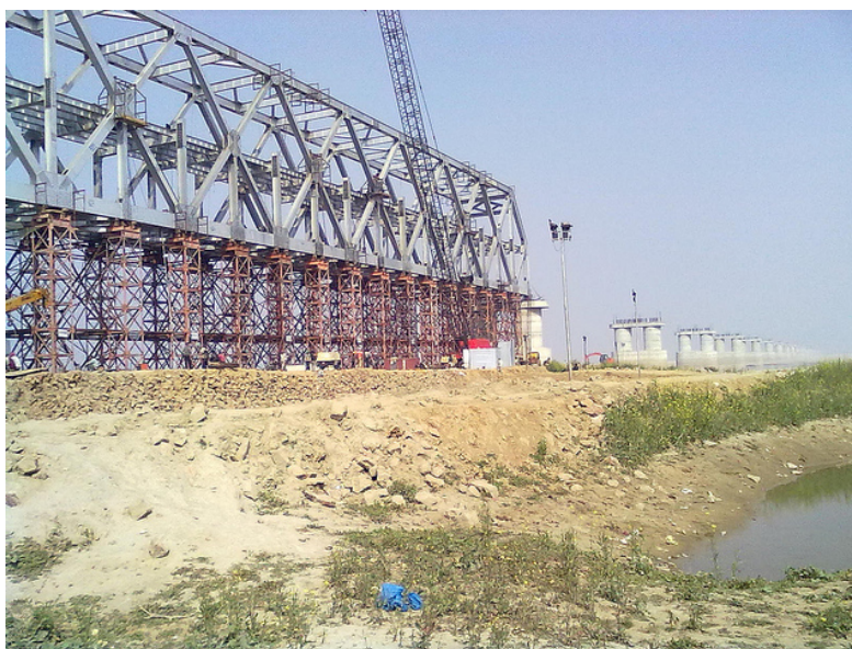
Ganga Bridge under construction at Patna
