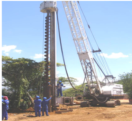
Bored Pile on a dry patch
