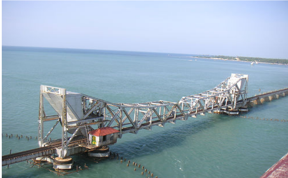
Pamban rail bridge –in closed position
