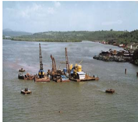
Pile driving in river
