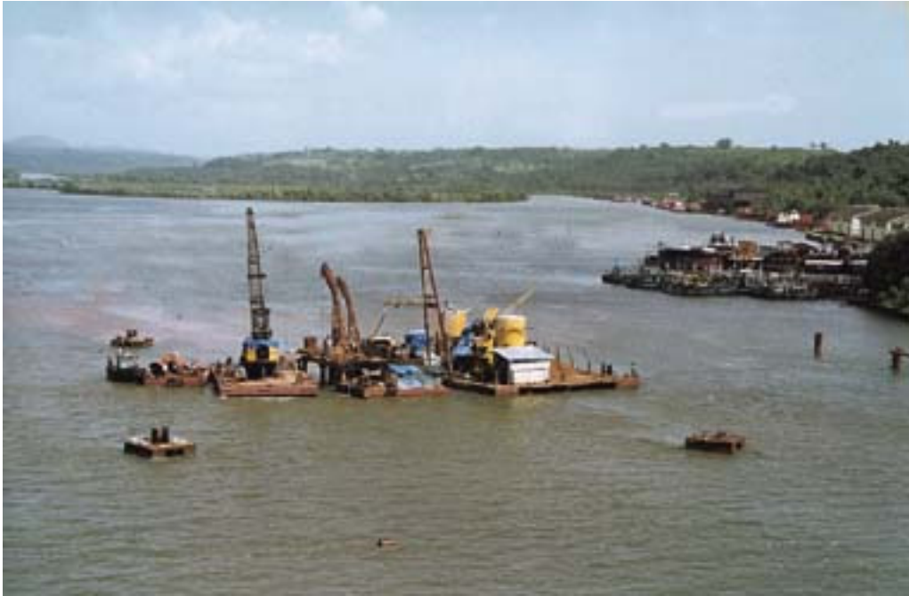
Well and Piling in progress
