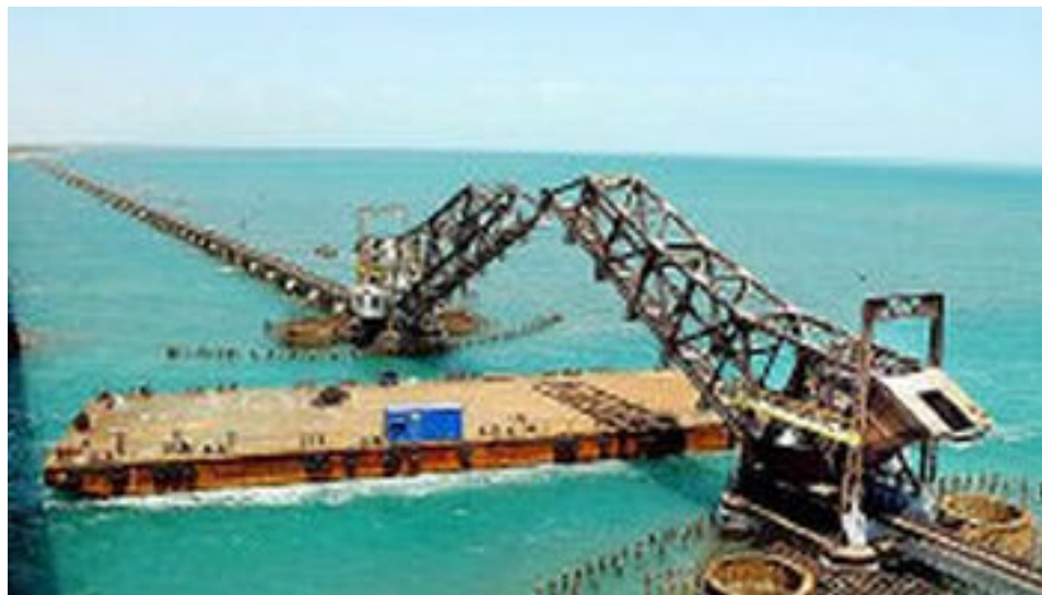
Pamban bridge –in open position to pass a vessel
