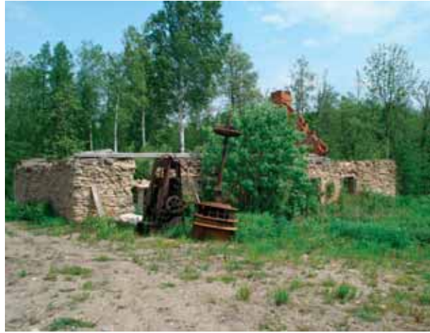
The ruins of the Iiba watermill are the silent witness of the glorious times of using hydropower. Photo: Aili Reiman.
