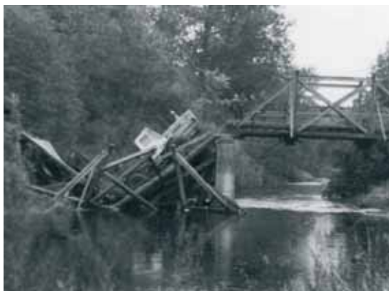
The old manor bridge in Tudulinna collapsed at the end of the summer of 1975, when a Kirovets K 150 tractor, of the then agricultural cooperative, was heading to the Tudulinna peat bog near the Suvajõe farmstead to pile peat. At that time, the Avinurme–Iisaku road passed through the small town of Tudulinna and across the old bridge. Photo: Mango Maasik.
