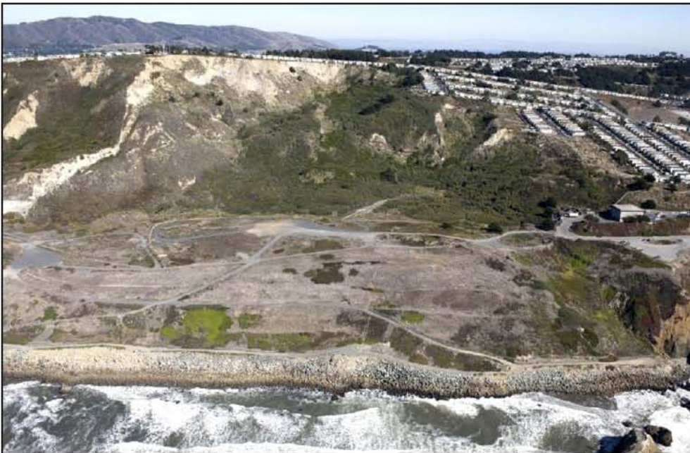
Figure 5. Main landfill pit and riprap apron fronting beach. From Adelman and Adelman (2009).
