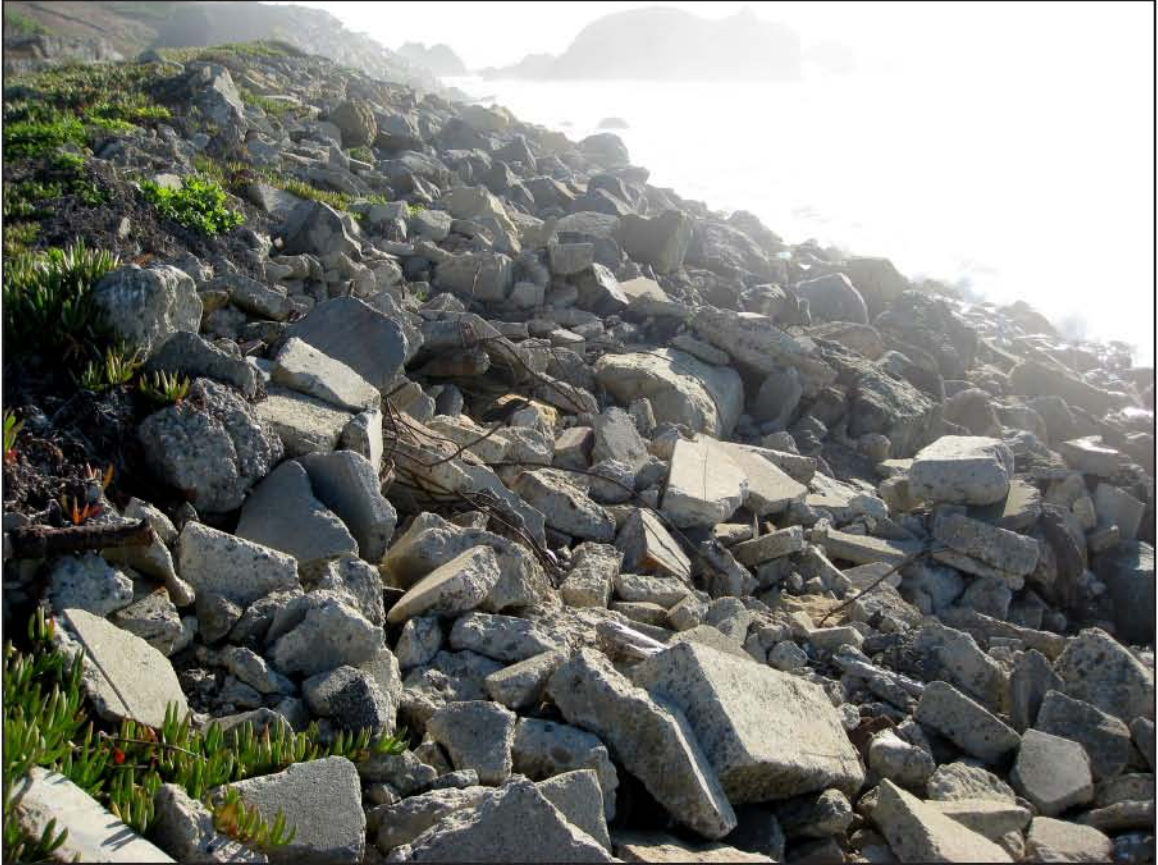
Figure 36. Riprap apron fronting landfill and covering beach, along with rebar and other detritus. Mussel Rock is in the background. Photo by Shawn Heiser.
