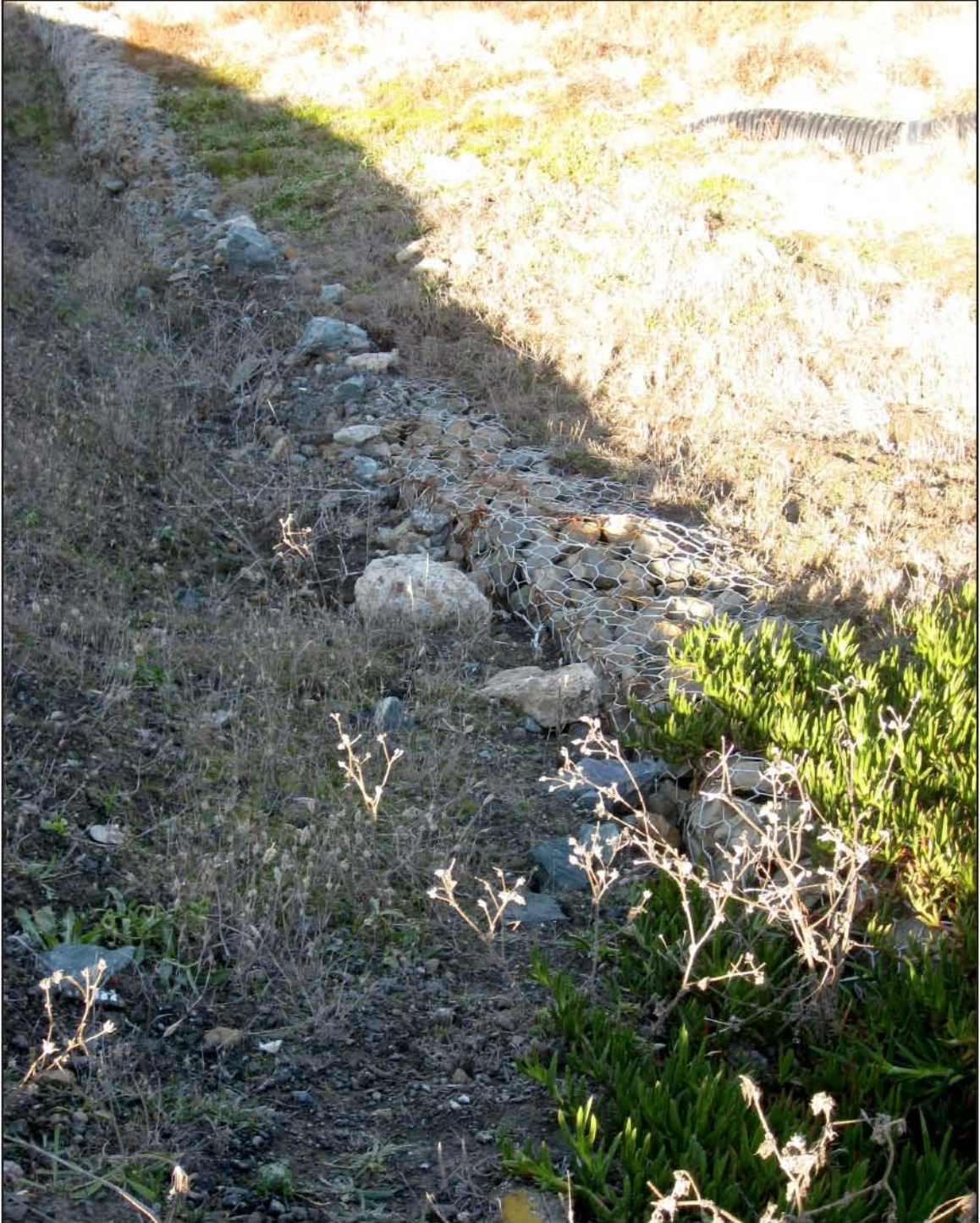
Figure 39. Relict seawall from 1965, nearly buried by fill and slump material. Photo by Shawn Heiser.
