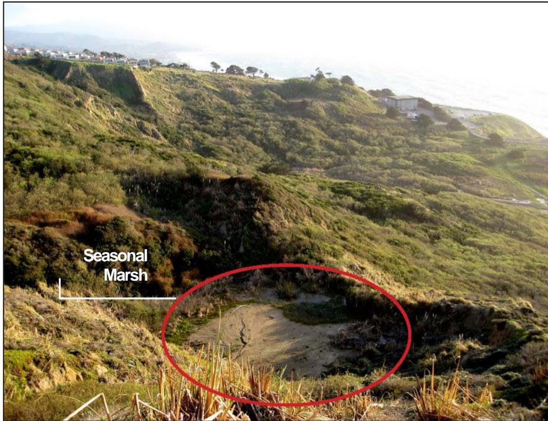
Figure 14. San Andreas Rift Zone and Mussel Rock Landslide, looking southwest. Seasonal marsh at bottom in Spring 2009. Note green space near top of photo where 21 houses have been removed due to landslides. Photo by Shawn Heiser.
