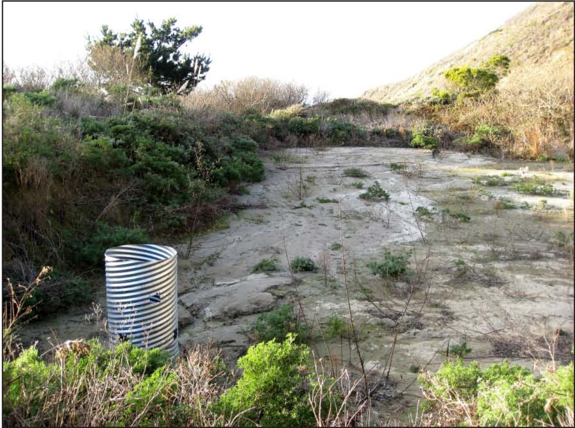
Figure 34. Upper North Canyon Landfill pit. Photo by Shawn Heiser.
