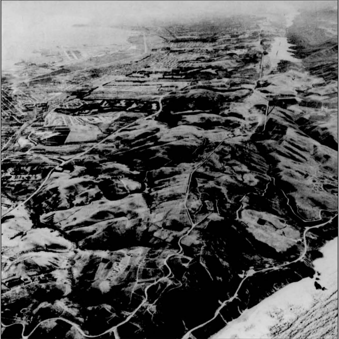
Figure 24. Aerial photo of the Sand Hills/Mussel Rock area from 1951, looking Southeast. Mussel Rock is at bottom right, below Ocean Shore Highway constructed along former Ocean Shore Railroad bed. Compare with Figure 32 (see page 90) to see subsequent development. From Cox-Whitsel (1983).
