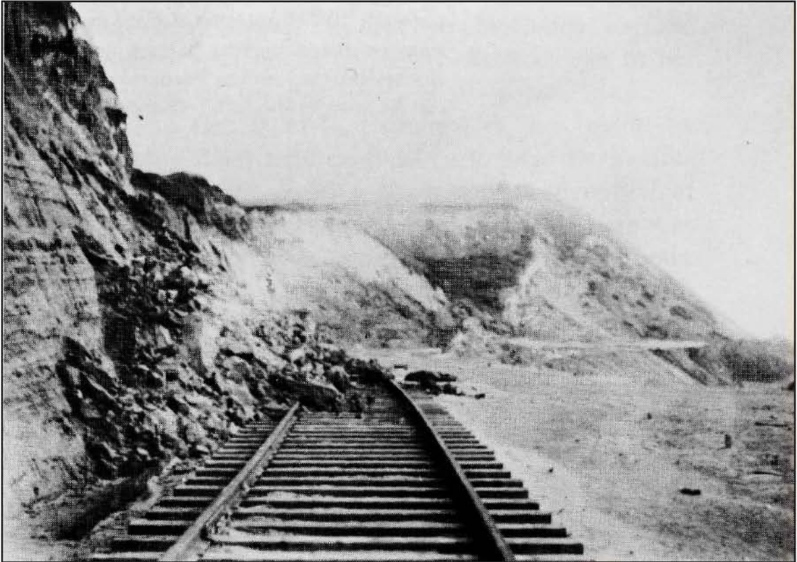
Figure 28. Landslide debris on Ocean Shore Railroad tracks following the 1906 San Francisco earthquake. From Wagner (1974).
