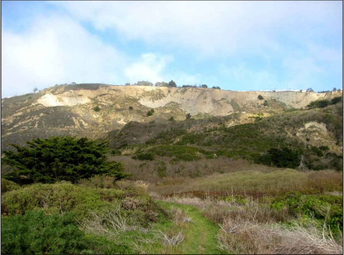
Figure 16. Northern and Eastern crown of the Mussel Rock Landslide, with residential homes atop the crown. Photo by Shawn Heiser.
