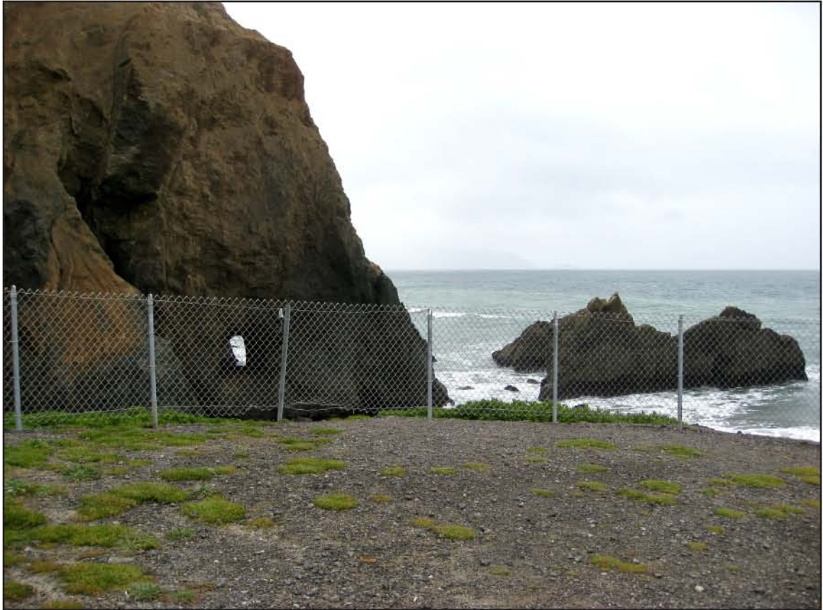
Figure 27. Fencing installed in 2008 to prevent access to Tobin's Tunnel. Portions of the fence have since been cut. Photo by Shawn Heiser.
