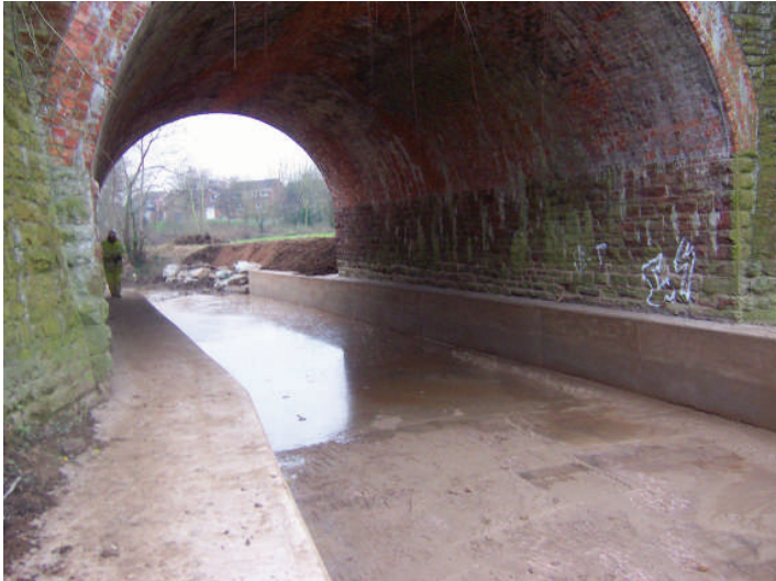
The saddle under the former railway arch
