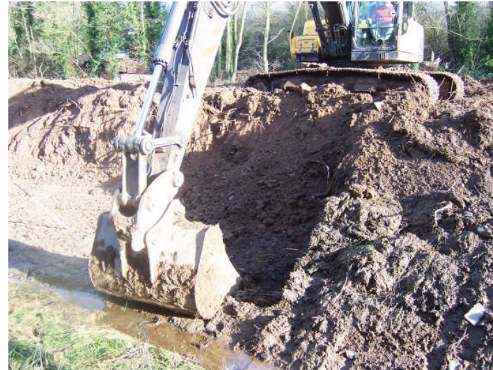
Cutting back of the bank of the mill stream
