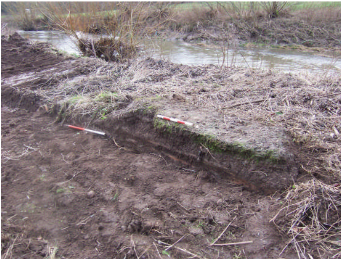
The brick and concrete cap over the sluice, with the Rea Brook in the background
