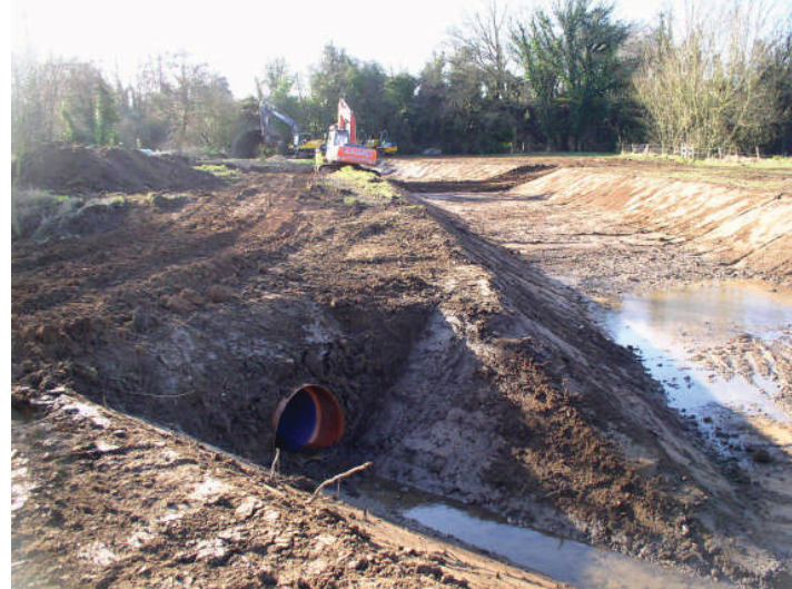
The new channel north of the railway bridge (looking south)
