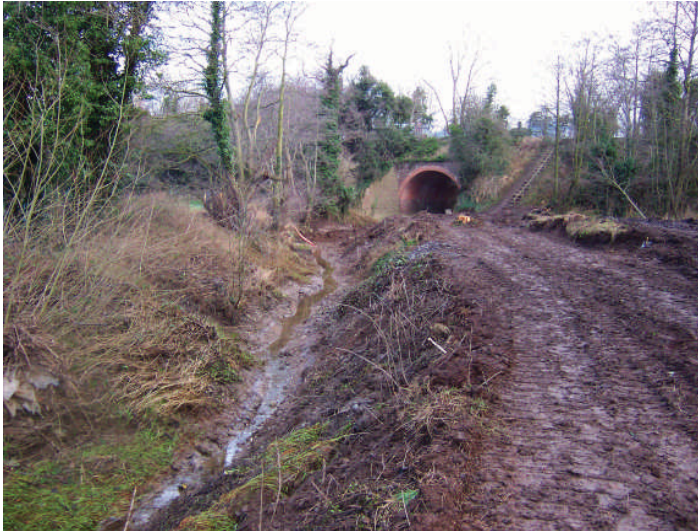
The mill stream, looking north, before widening
