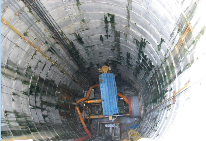
• A confined shaft
