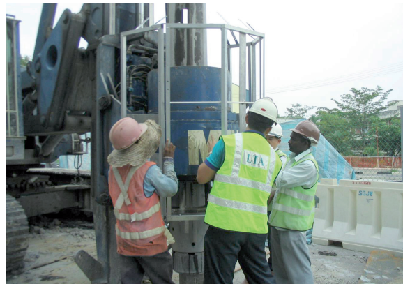
• Mounting of aluminium frame on rotary head
