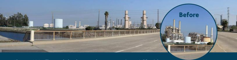
The new AEC will not only be cleaner and more responsive to California's energy needs, the new plant will also be shorter and sleeker, reducing visual impact and improving its appearance for local neighbors. Currently, the tallest structure at the existing plant is about 214' - the tallest structure at AEC will be 150'.
