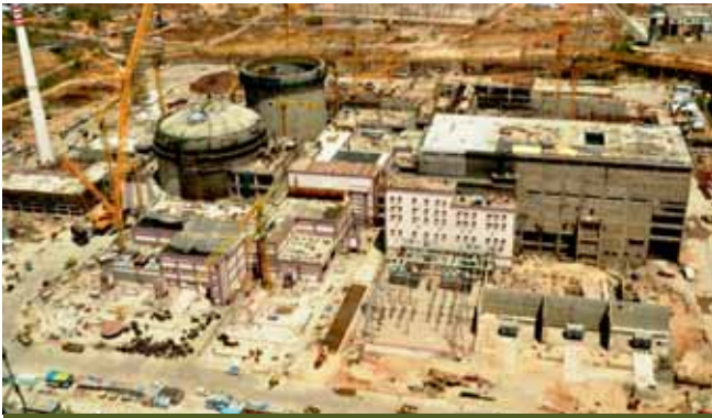
Main Construction area of RAPP-7&8
