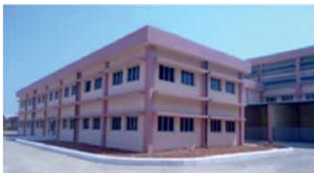
MRTDDF - Office Building
