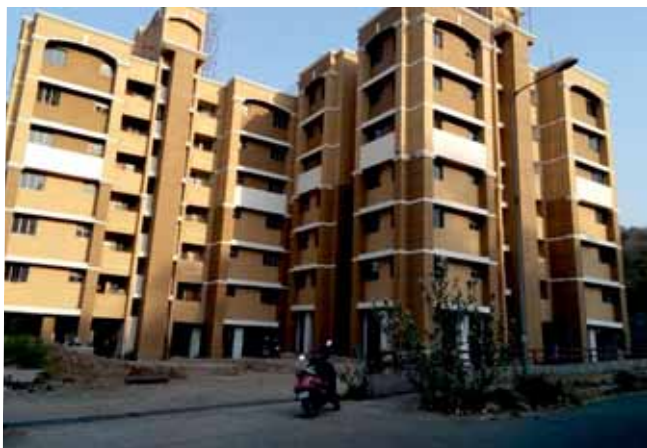
Residential Quarters at Anushaktinagar, Mumbai
