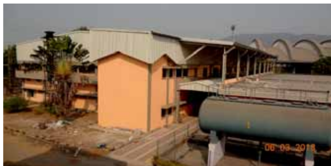
Construction of Advanced Radiation Technology Laboratories for RPL, BRIT at Vashi, Navi Mumbai
