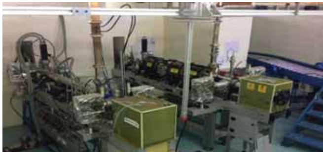
Linac-B1 and Linac-B2 installed at radiation processing facility
