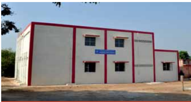
Construction of Girls Hostel at Ghata, Kakrapar site
