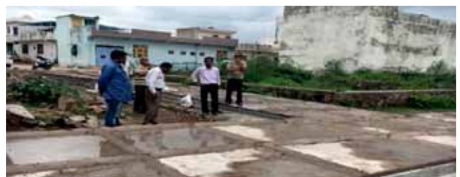
Cement concrete link road at Rawatbhata site
