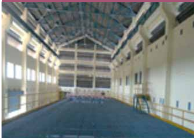
MRTDDF - Cell Building
