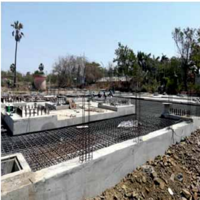
Construction Civil Work at R&D Centre
