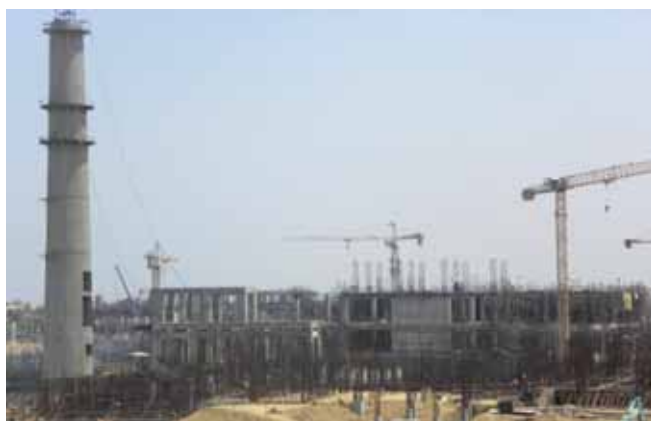
Overall view of FRFCF site under construction
