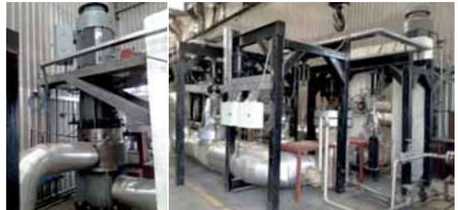
700 MWe Shutdown Cooling Pump and Test Loop erected for Endurance Test
