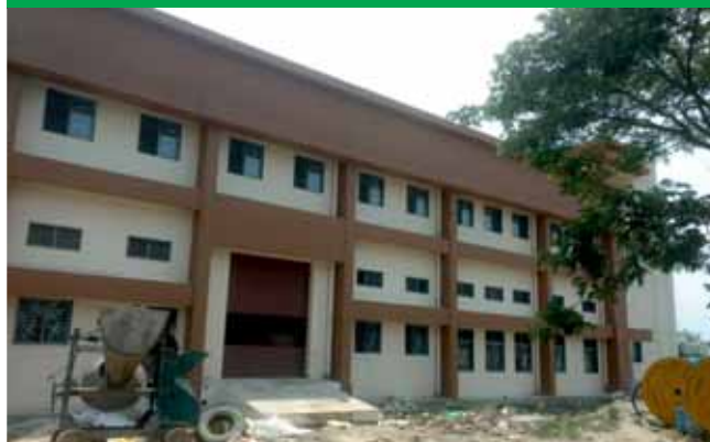
Construction of Electrical Substation at Rajarhat, Kolkata
