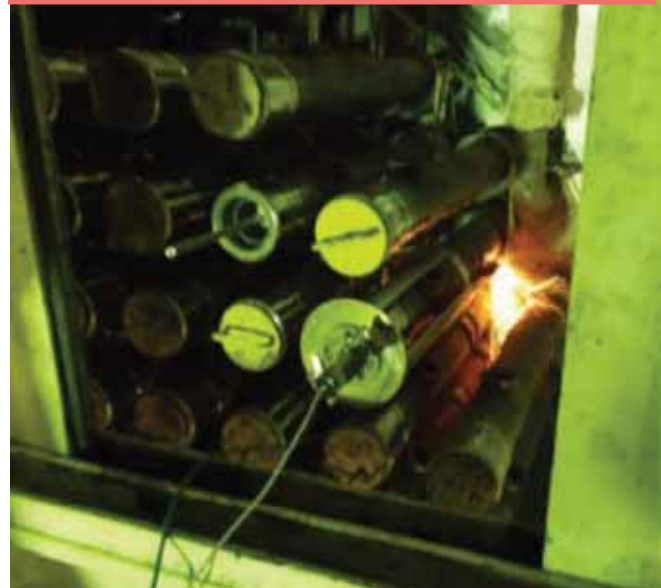
In-situ laser cutting of bellow lip weld joint in KAPS-1 reactor
