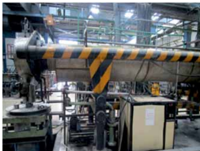
Installation and commissioning of 2TR chiller in Stabilization Unit
