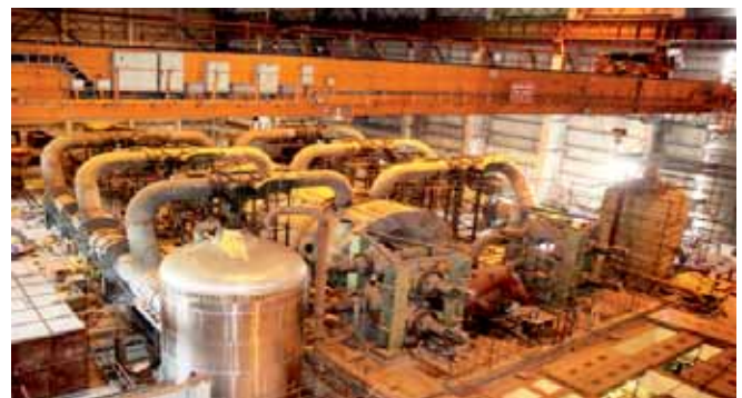
High Pressure and Low Pressure Turbine box-up at KAPP-3
