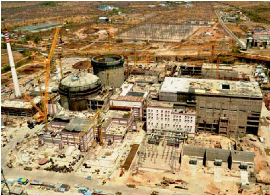
Main Construction area of Rajasthan Atomic Power Project (RAPP) Unit-7&8
