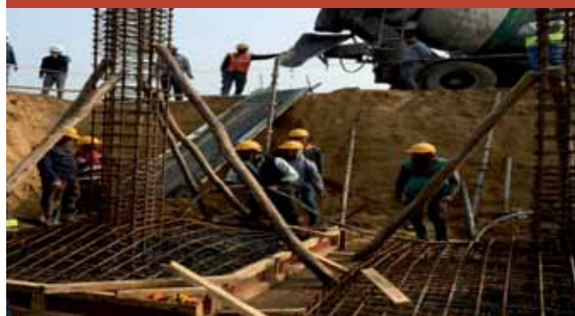
Concrete pouring at Residential Complex
