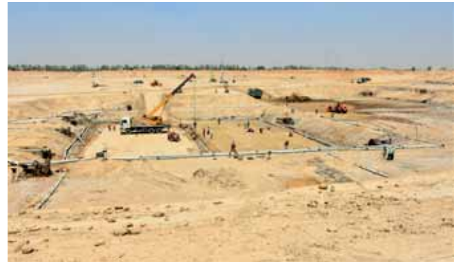
Ground improvement works at GHAVP Unit-1&2
