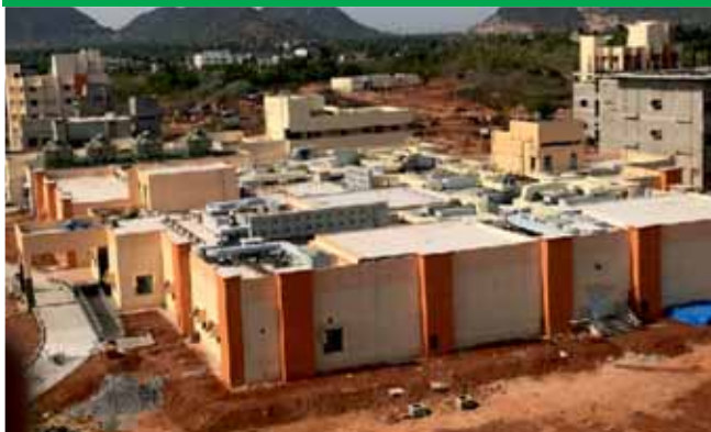
Radio Therapy Block of 100 Bedded Hospital Complex at Visakhapatnam, Andhra Pradesh
