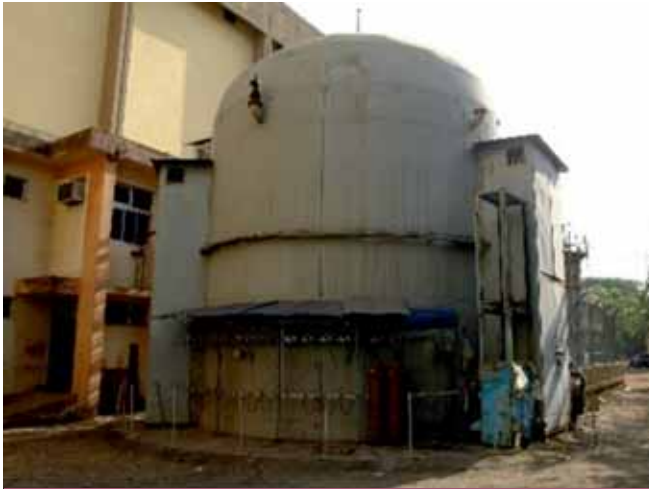
Containment Study Facility at Hall-7, BARC (Schematic and Actual)
