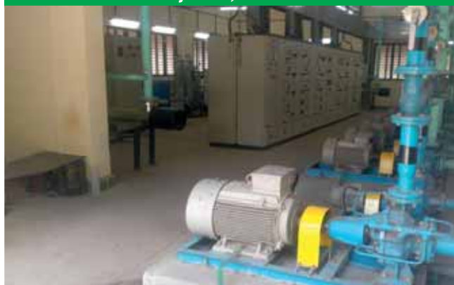
Construction of Ancillary Structure for Sewage Treatment Plant at Anushakthinagar, Mumbai
