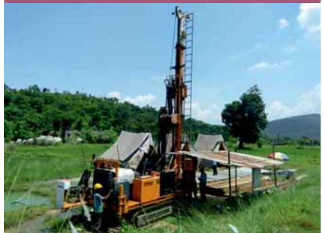
Newly procured hydrostatic core drilling rig (KDR-600) in operation at Kudada area, East Singhbhum district, Jharkhand
