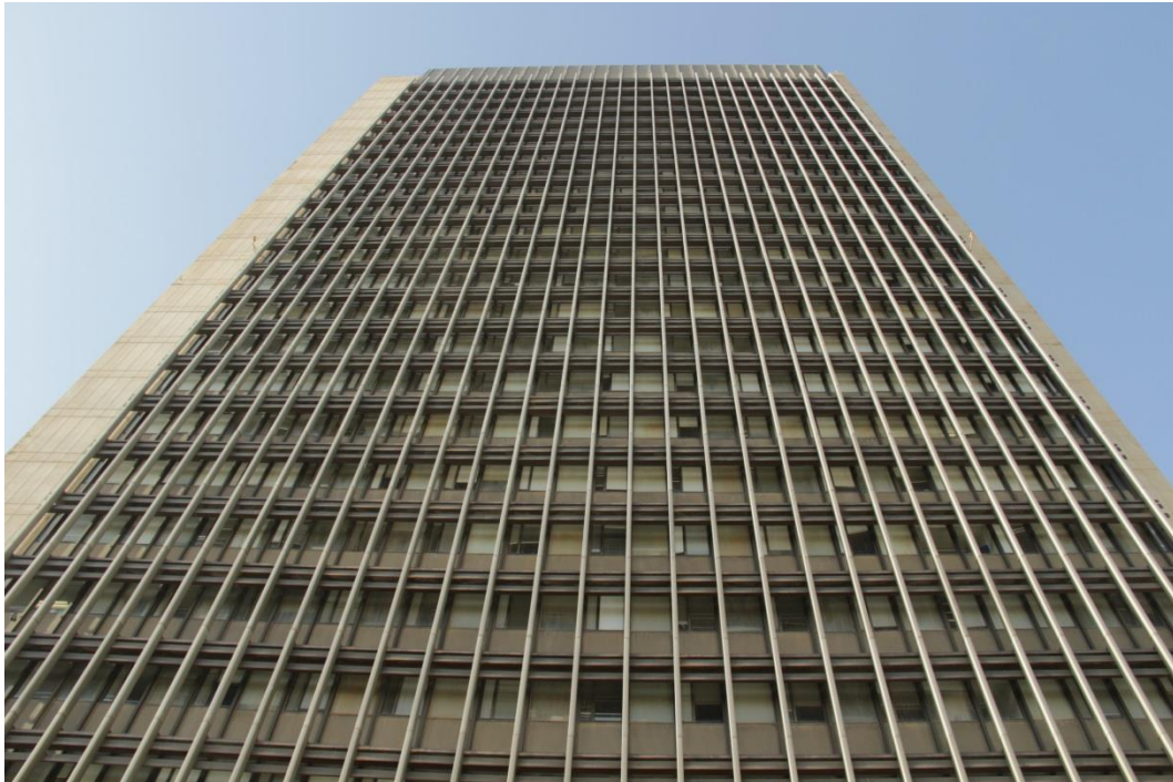
Figure 6.35: Eshkol Tower, the south-eastern facade, December 2013, showing the extensive use of venetian blinds in the rooms (photograph by the author).
