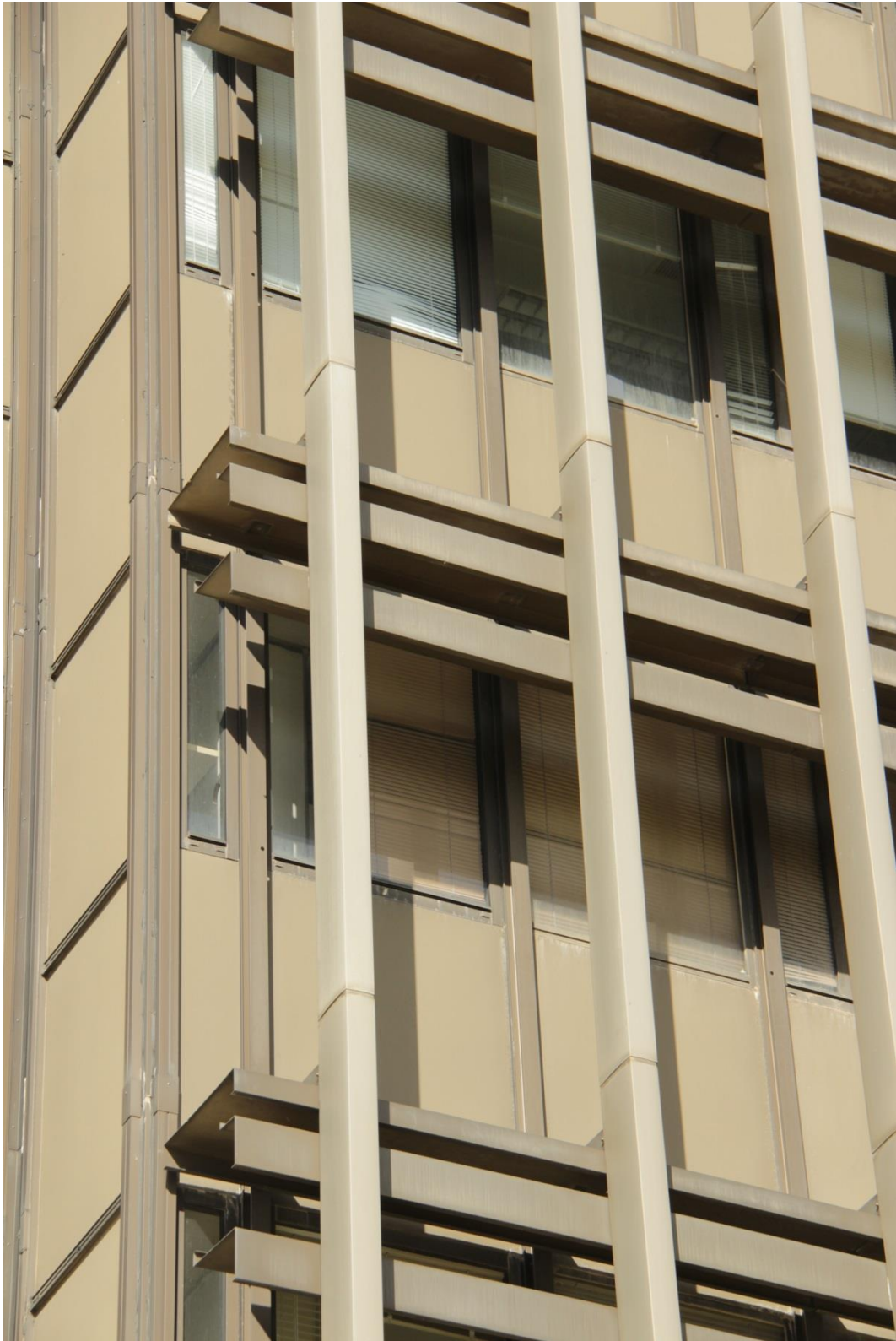
Figure 6.33: Eshkol Tower, the sun breakers system as realized, the south-eastern facade, 2013 (photograph by the author)
