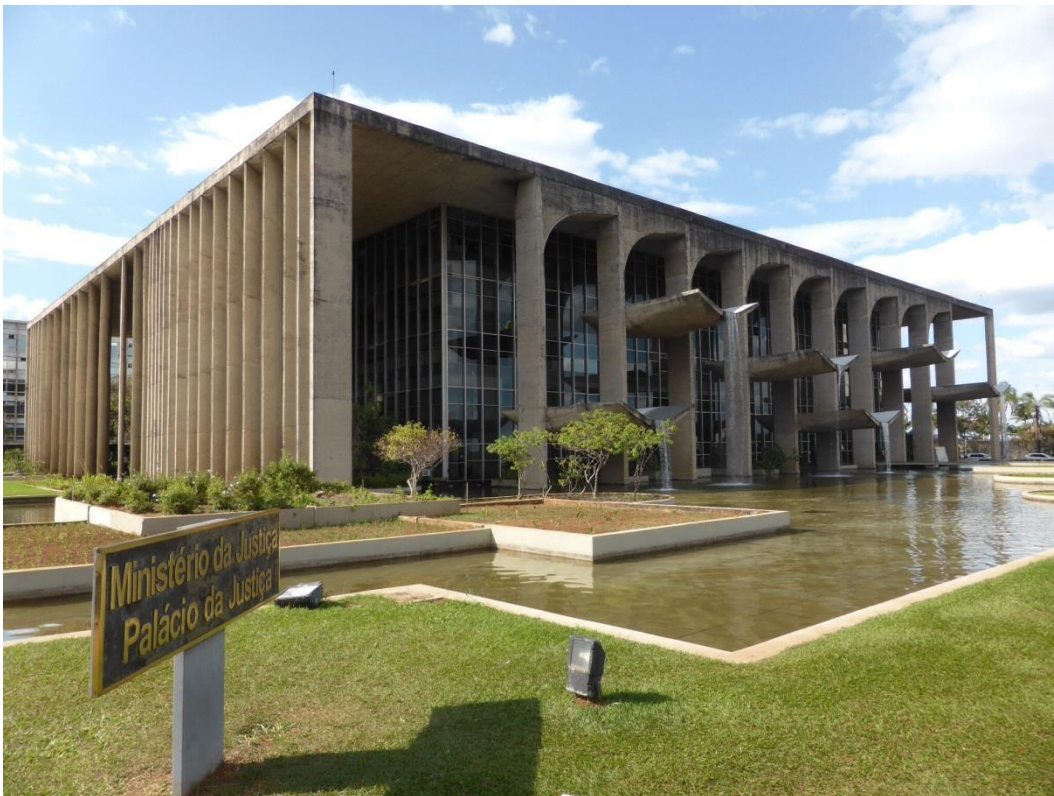
Figure 6.24: Oscar Niemeyer, the Ministry of Justice Building in Brasília, 2014 ( https://goo.gl/HxTzN5 ). The diagonal sun breakers of the north-western facade are seen to the left
