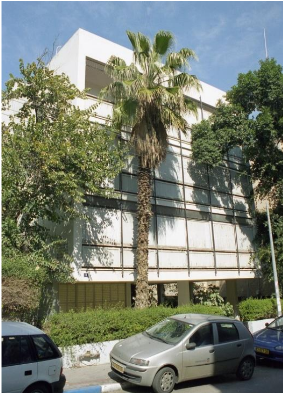
Figure 4.22: Dov Karmi and Hever Architects, Orenstein House, 3 Rosenbaum Street, Tel Aviv, 1955 (photograph by the author, 2003). The facade to the street is covered with slatted shutters, of which the bigger panels are sliding one behind the other and the smaller panels are fixed and used as railings
