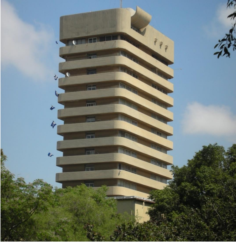
Figure 6.37: Moshe and Mordechai Ben Horin, Metzudat Ze'ev office building in Tel Aviv (1963-1965), 2011 (photograph by Yoav Lerman)
