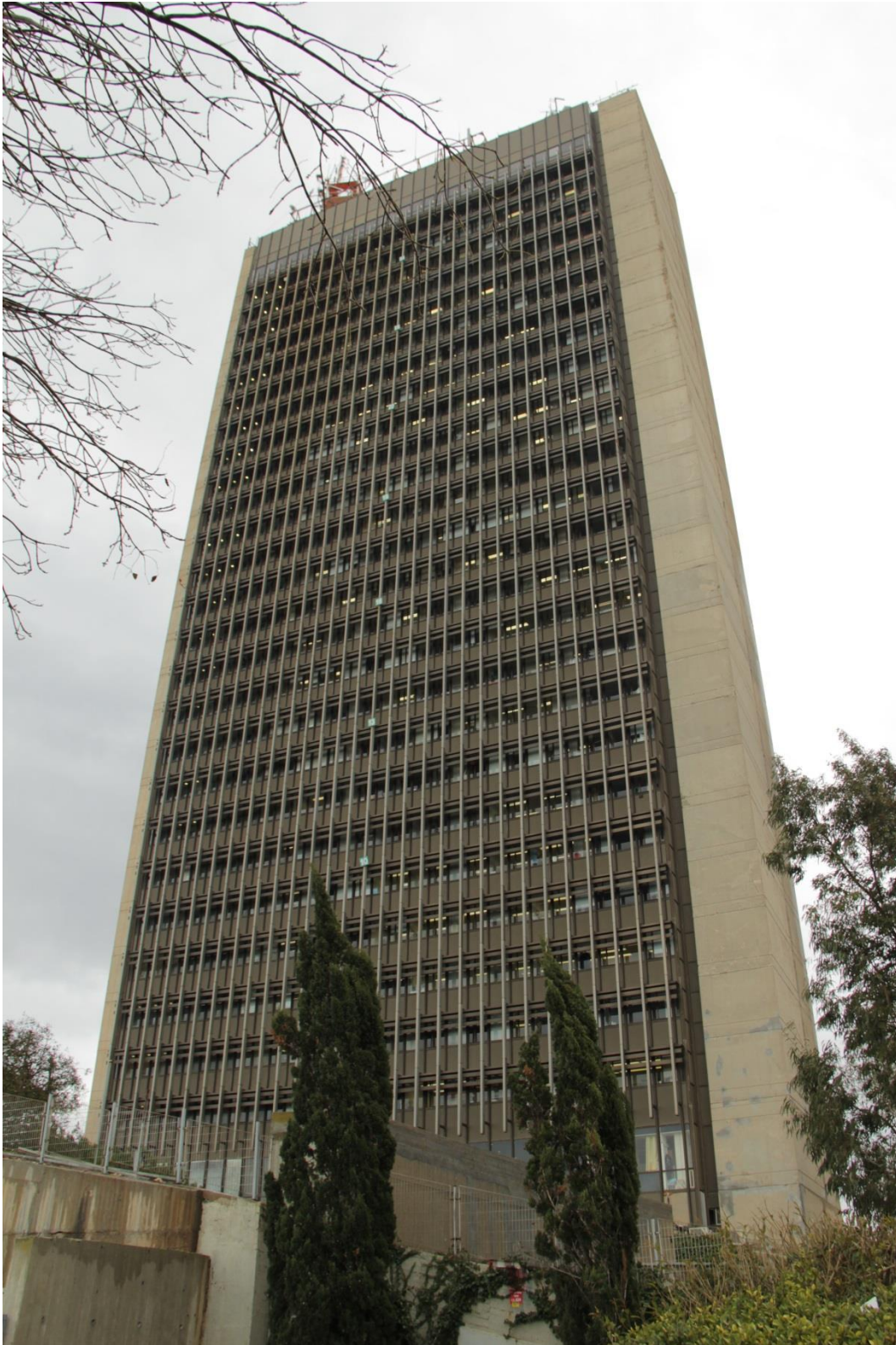
Figure 6.34: Eshkol Tower, the north-western facade, 2013, showing the realized sun breakers system in its full extent (photograph by the author). Identical sun breakers were installed also on the south-eastern facade
