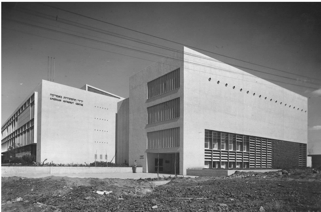
Figure 4.8: Arieh Sharon and Benjamin Idelson, the southern and western facades of Hamlin House and the western facade of Lessin House, Tel Aviv, 1956 ( www.ariesharon.org )
