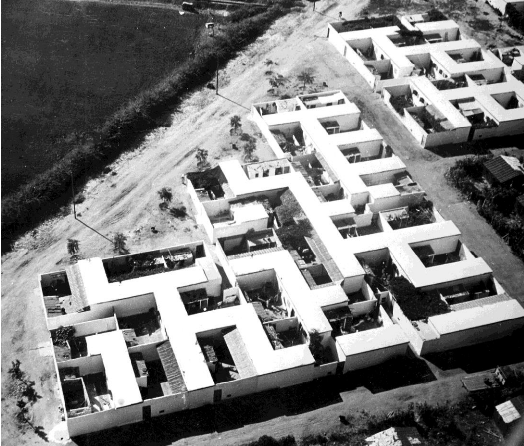
Figure 5.24: A group of realized housing units built according to the Écochard grid system in Yacoub El-Mansour quarter in Rabat, 1954 (Michel Écochard Collection, Aga Khan Trust for Culture)
