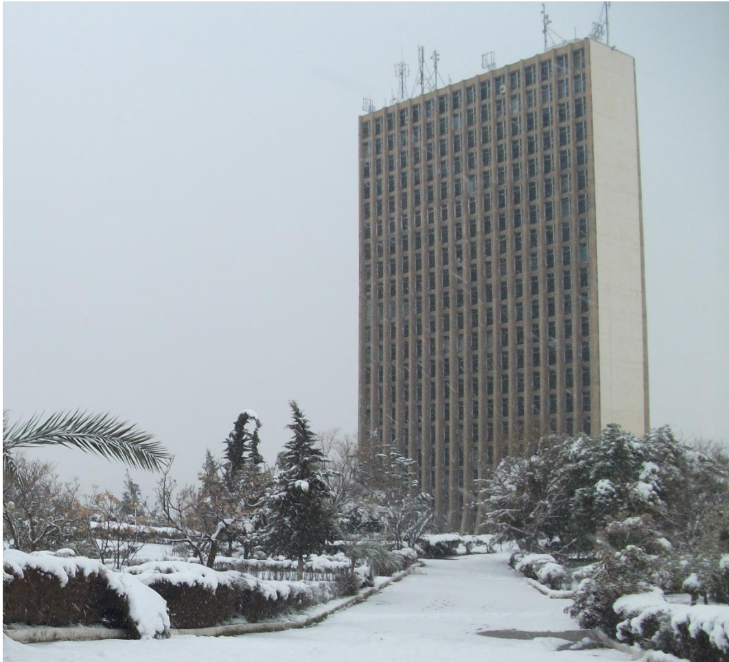
Figure 6.22: Oscar Niemeyer, the administration tower at the University of Mentouri, Constantine, southern facade (photograph by Mostafa MT, Panoramio)
