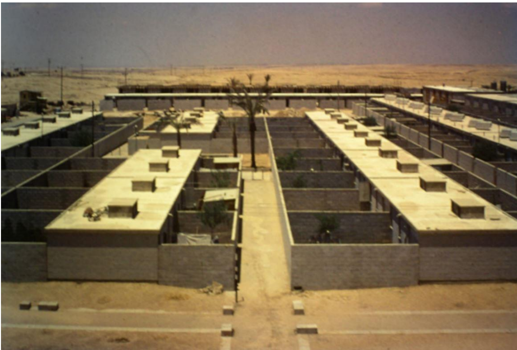
Figure 5.29: A rare colour slide of the carpet housing showing houses of types A and C, photograph by architect Daniel Havkin (Havkin Collection, Israel Architecture Archive). The whitewash of the roofs is clearly noticeable, as well as the non-whitewashed walls
