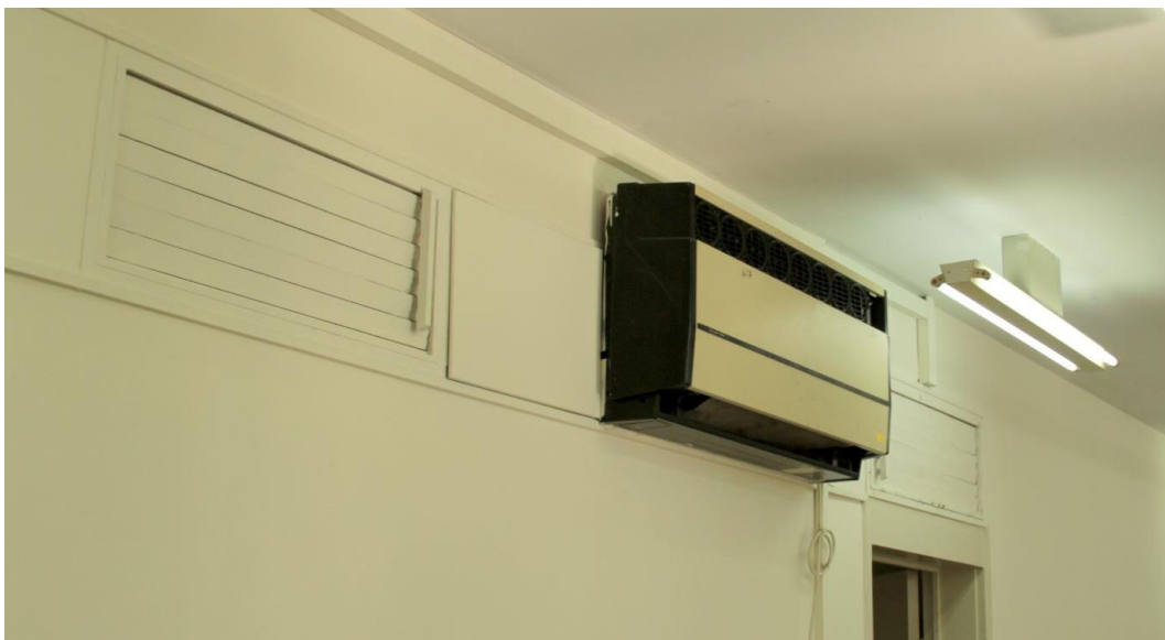
Figure 4.49: Rare original ventilation shutters, now unused, inside a classroom in the Gilman Building, leading to the air space above the adjacent corridor that connects to the facade to the courtyard, 2014 (photograph by the author)
