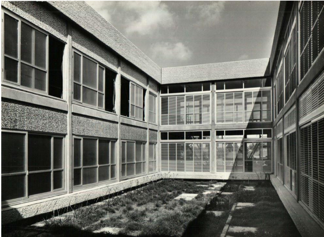
Figure 4.43: Gilman Building, the smaller courtyard of the southern wing, looking east, ca. 1966 (Israel Stein Collection). The corridor facades, here facing north and west, were screened with sliding aluminium panels of rotatable PVC slats
