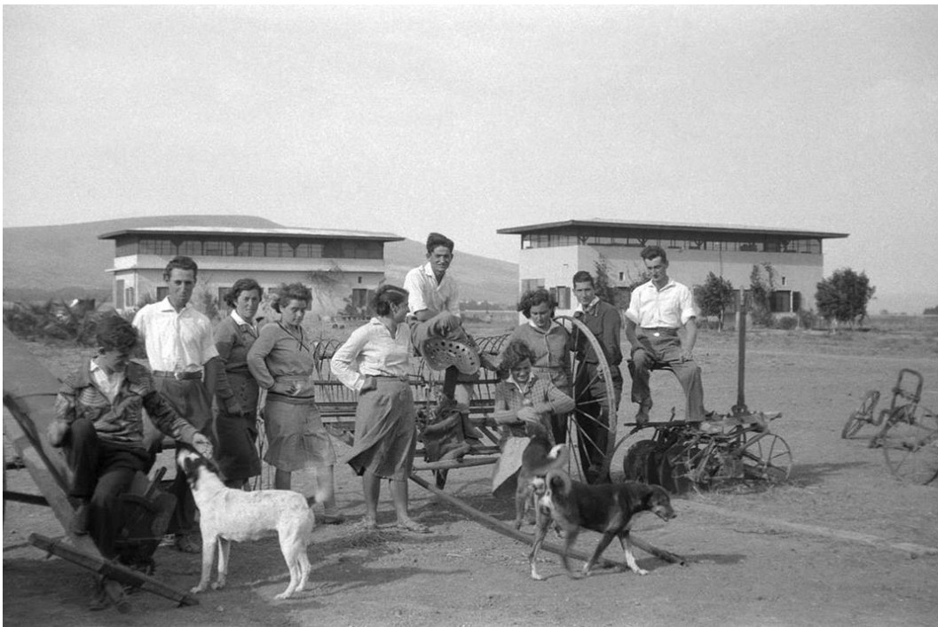
Figure 2.1: Richard Kaufmann, residential buildings in Kibbutz Beit Zera with "double roof" consisting of light roofs shading over the structural concrete roofs, 1932 (photograph by Ze'ev Aleksandrowicz)
