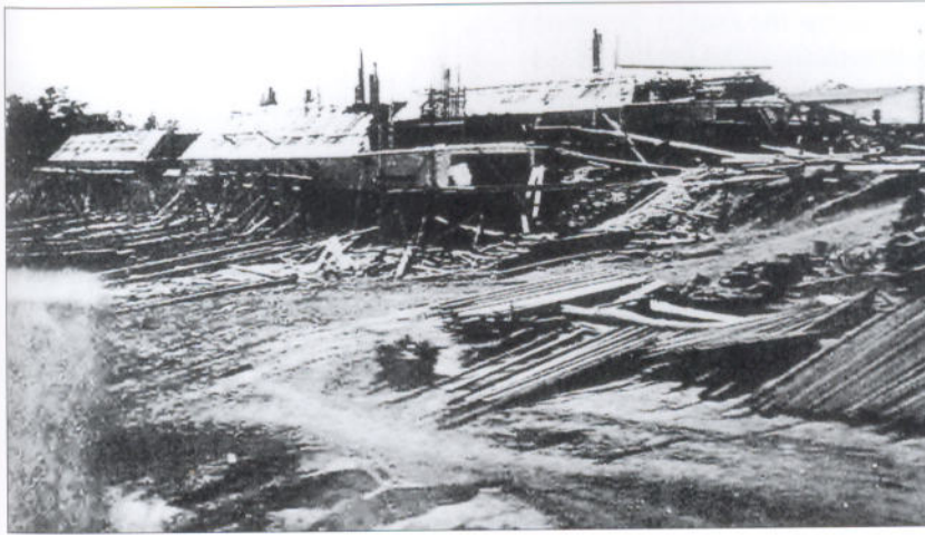
The building of a City class ironclad at Carondolet, Missouri. Four vessels can be seen, on two levels, facing bow to bow. All seem to be in a roughly similar stage of construction. Once finished, the ironclads would be launched sideways down the "marine ways" or runners leading to the Mississippi River, just to the left of the cameraman. (USNHC)
