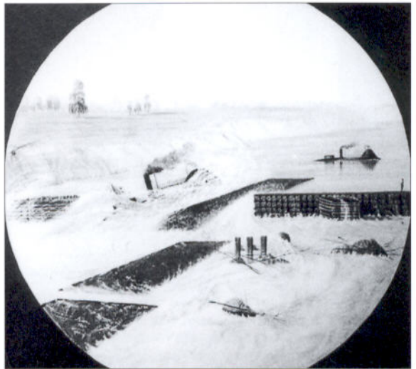
The USS Osage and USS Neosho depicted running through a gap in the Red River Dam near Alexandria, Arkansas, on May 9, 1864. The passage took advantage of an accidental break in the dam, which had been built by the Army to raise the river level and so rescue the Union warships trapped on the Red River. Watercolor by James Alden. (USNHC)
