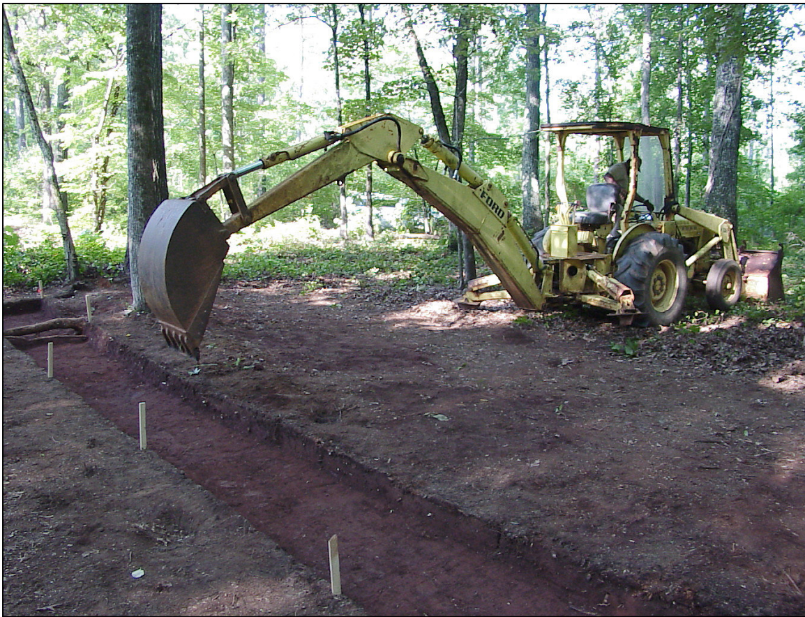
Figure 17. Backhoe Excavations.
