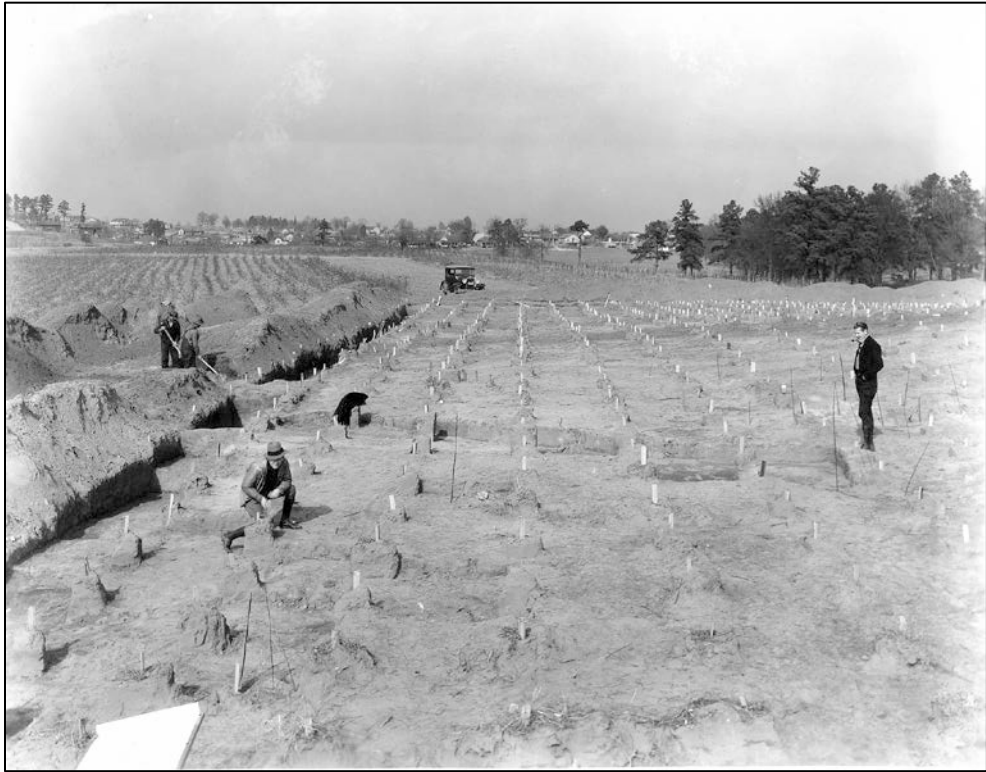
Plate 1: Clearing of Mound Surface from West Baseline
