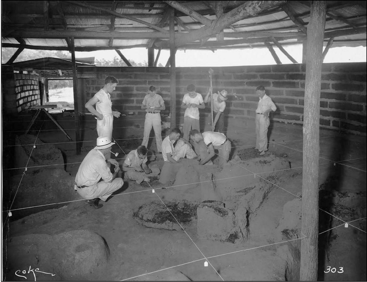
Plate 38: Students Removing Timbers from Council Chamber
