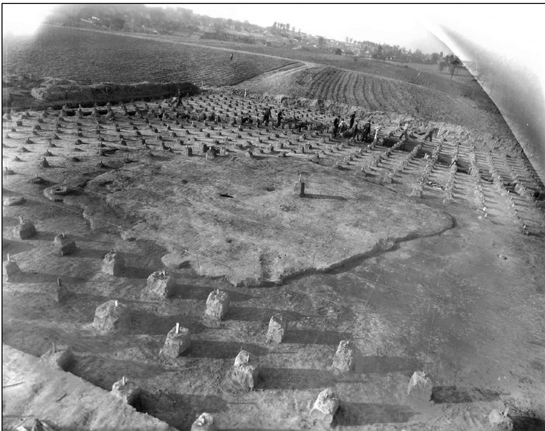
Plate 3: Initial Clearing of Clay Platform on top of Mound D
