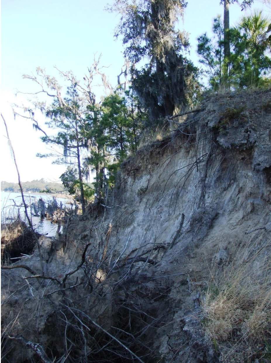
Figure 7. Bank Erosion of Rose Dhu Battery at Rooster Point, 2010.
