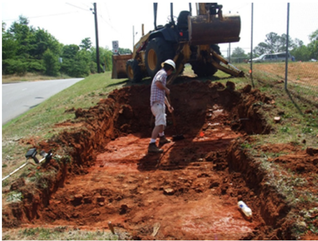
Figure 8. Joel Jones Monitors Progress of Backhoe Excavation Unit 27, East View.
