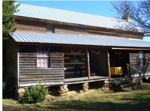
Figure 5. Rear View of Fort Hollingsworth, 9BA7, Facing Southwest (Beavers 2012).
