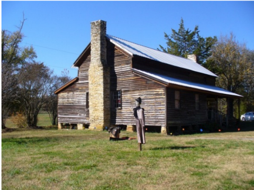
Figure 4. Rear View of Fort Hollingsworth, 9BA7, Facing Southwest (Beavers 2012).
