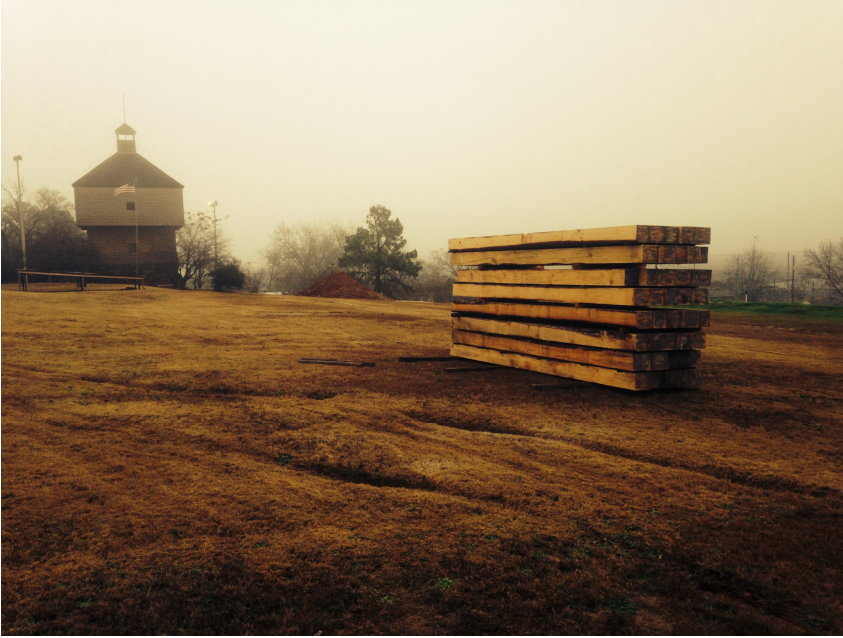
Figure 11. Logs Stockpiled for Reconstruction, December 2013.
