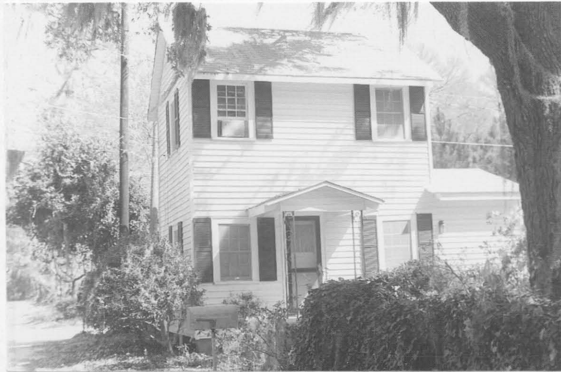
Figure 11. House at 731 Dancy Avenue.
