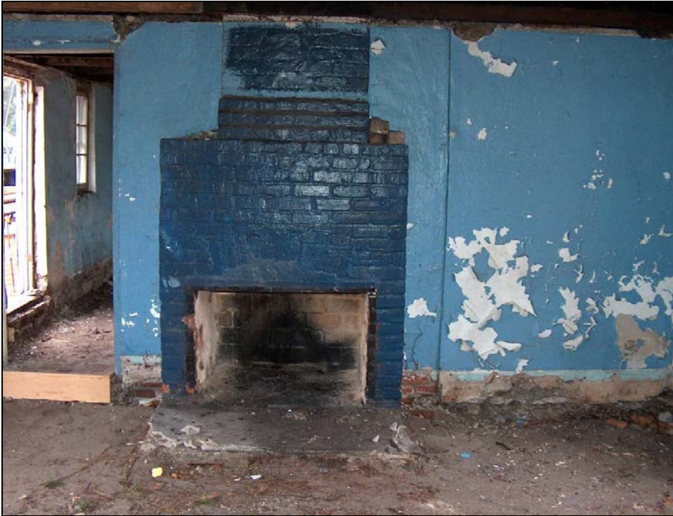
Figure 4. Interior View of a Tabby Duplex after Removal of the Flooring, 9Ch1062.
