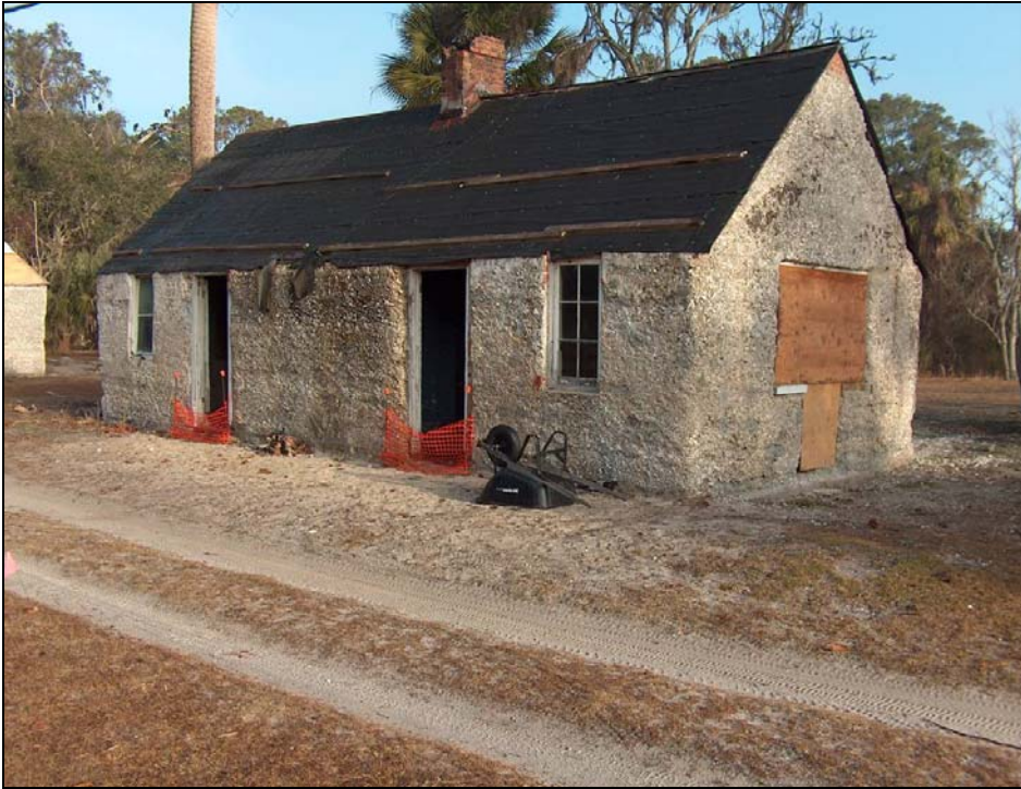
Figure 3. View of Tabby 1, Facing Northwest, 9Ch1062.
