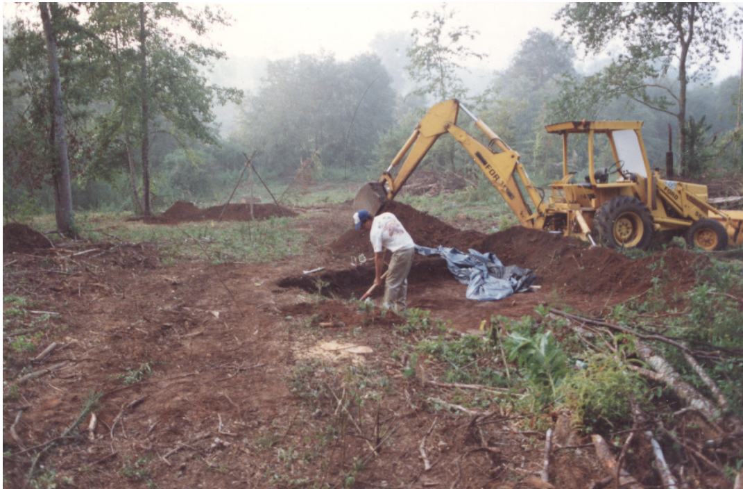
Figure 5. Excavation at 9HM176.
