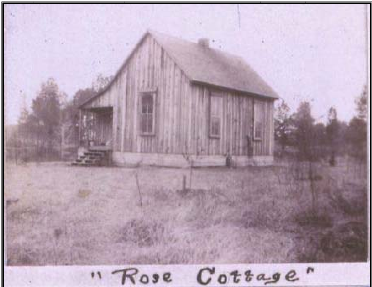
Figure 6. Rose Cottage (George Gibson house) at Commonwealth (note board and batten construction) (Courtesy, Hargrett Rare Book and Manuscript Library, University of Georgia).
