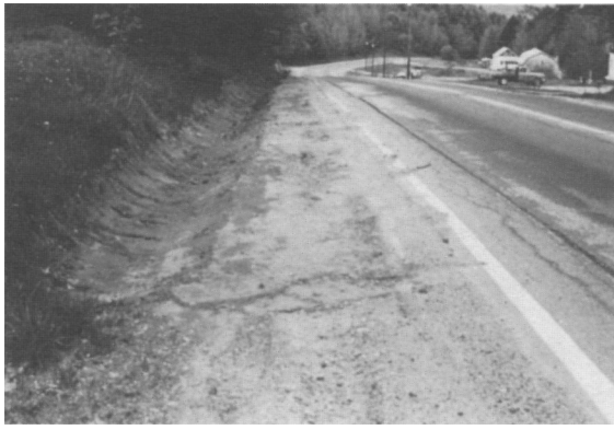
Good ditch and shoulder maintenance
