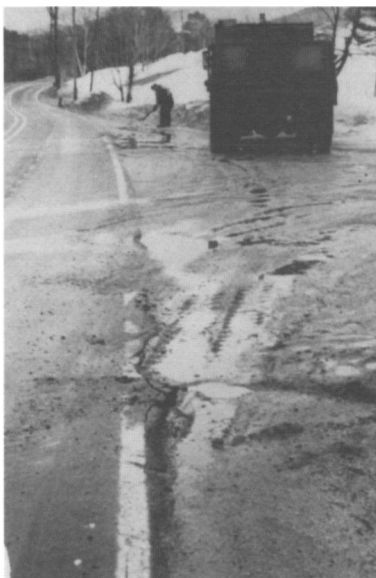
Clearing drainage to prevent edge failures
