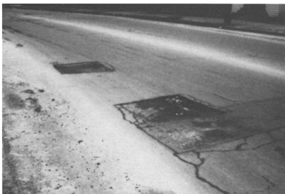
A good inspector can spot areas that need repair before a pothole develops
