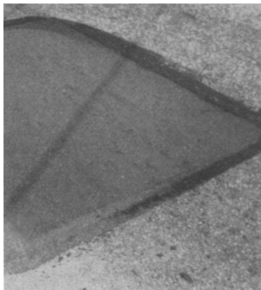
Edge sealing of patch (above) is an important detail that prevents early edge failure by intrusion of water
