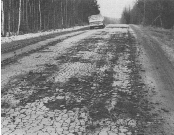
One harsh winter can destroy a poorly maintained road (Bangor Daily News)
