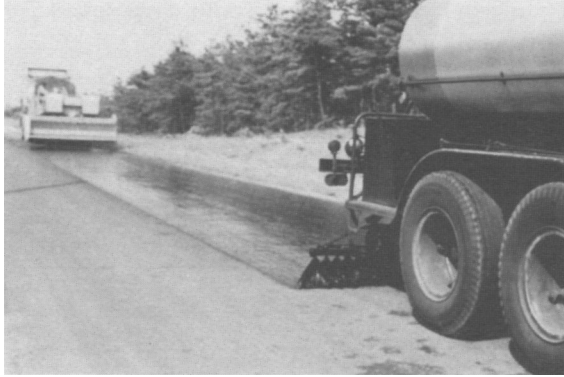
Periodic surface treatments seal out water
