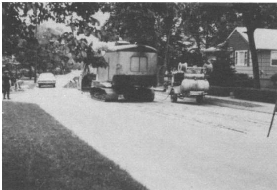
Utility cut operations should be coordinated with resurfacing
