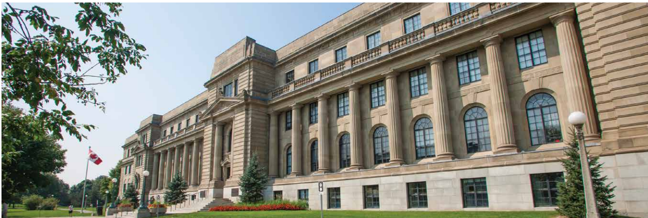
Figure 4.9: In 2012, the FBI program facilitated an energy retrofit project at the National Research Council building (100 Sussex Drive, Ottawa). An investment of $9 million dollars resulted in annual utility and maintenance savings of $920 thousand dollars.
