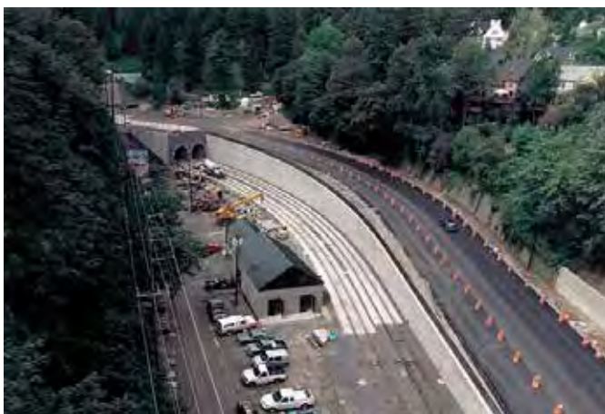
Westside MAX tunnel east portals, 1997
