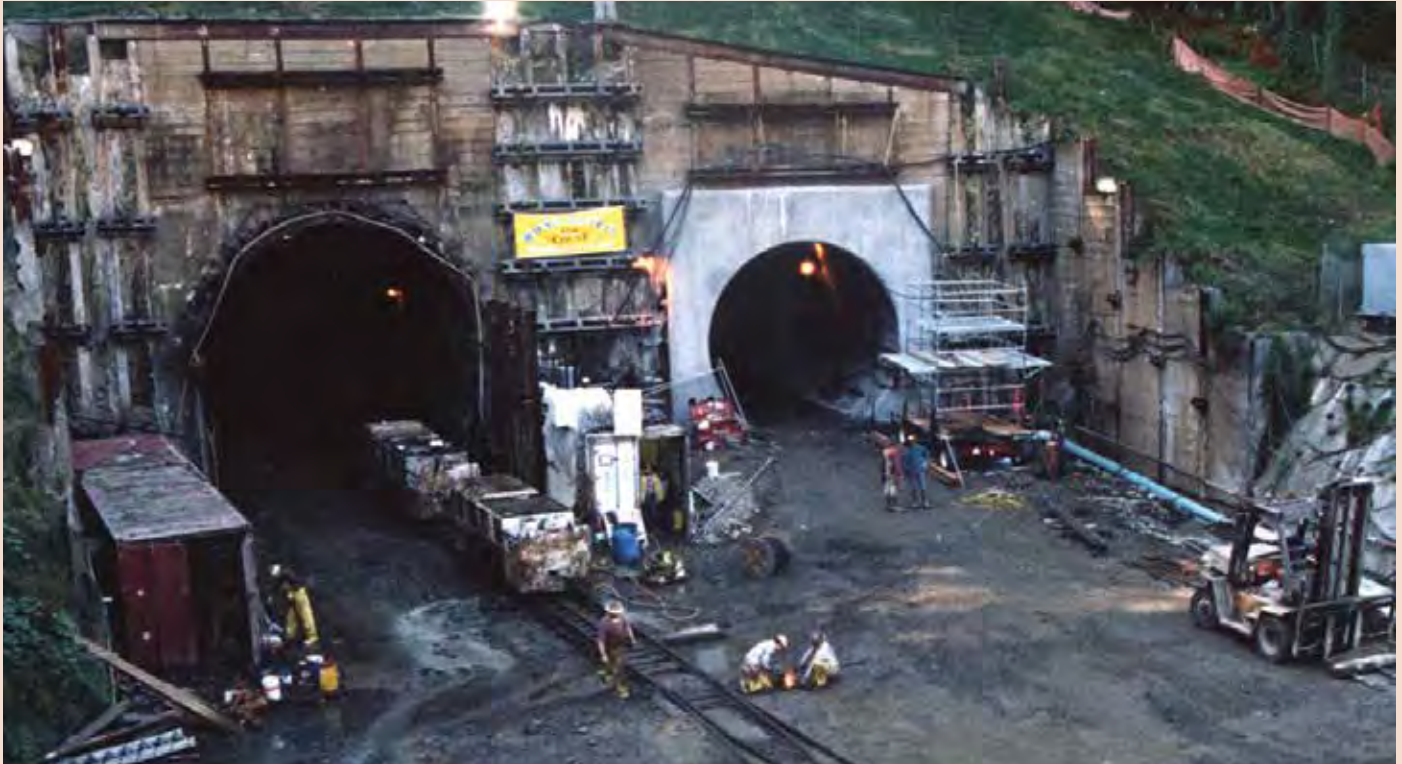
Westside MAX tunnel east portals, 1995
