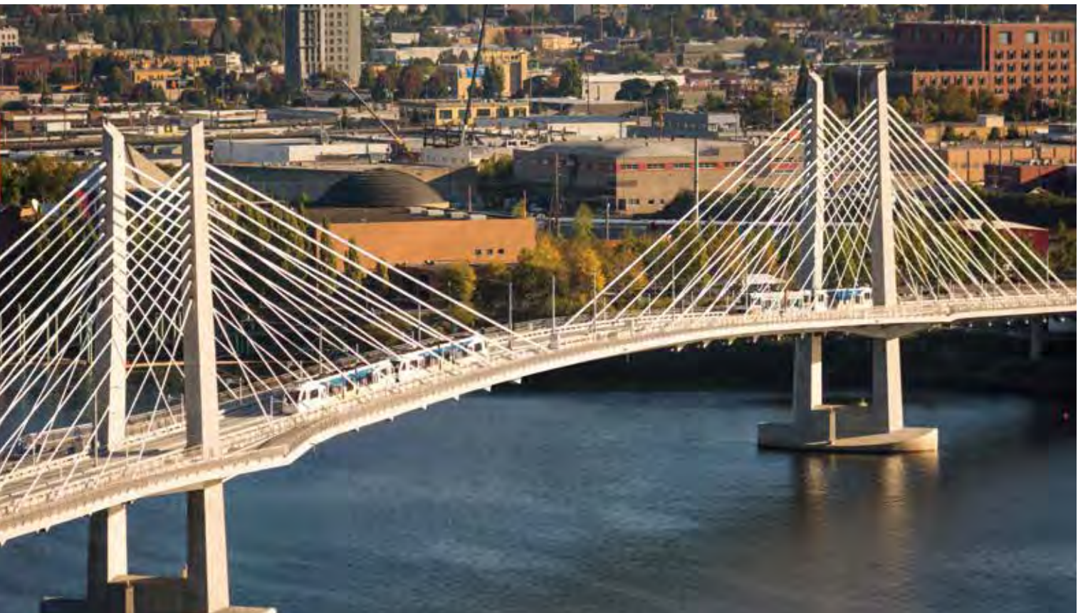
Tilikum Crossing, Bridge of the People , 2015
