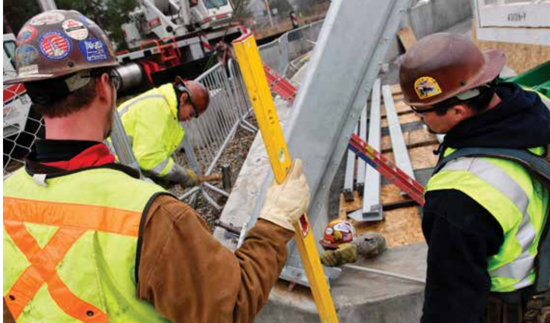
Construction workers on MAX Green Line, 2009
