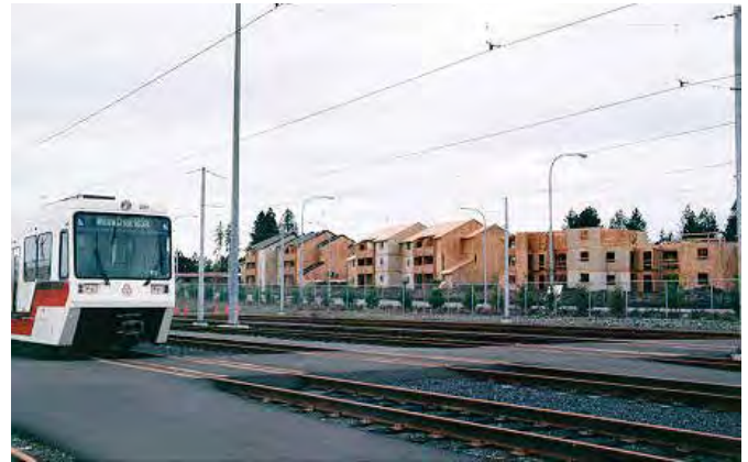
Gresham Central Apartments, a transit-oriented development in Gresham, 1996
