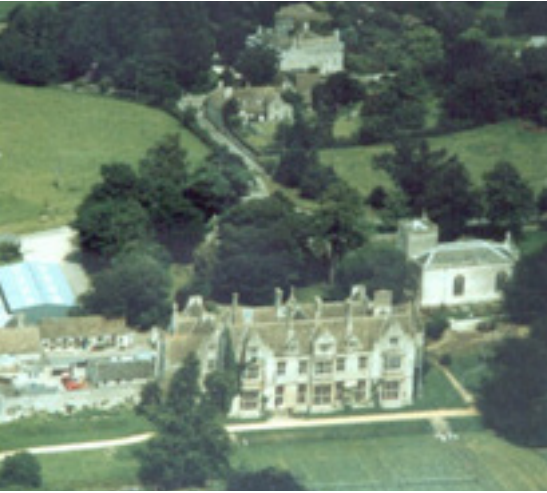
Alderley Manor, Gloucestershire
