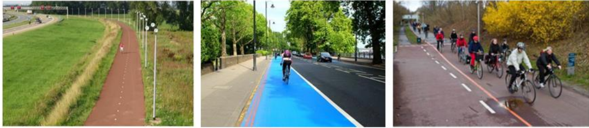
Figure 3.5 Examples of different executions of coloured surface. (Bicycle Dutch, 2015), (London Cyclist, 2011), (Sørensen, 2012)
