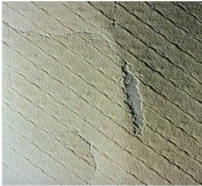
Figure 56. Picture of scaled membrane surface with imprints from the feed spacer
