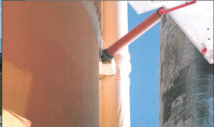
Left Bipod Foam Ramp where the loss of debris occurred on STS-107. Left side is the external tank, and right side is the orbiter.
