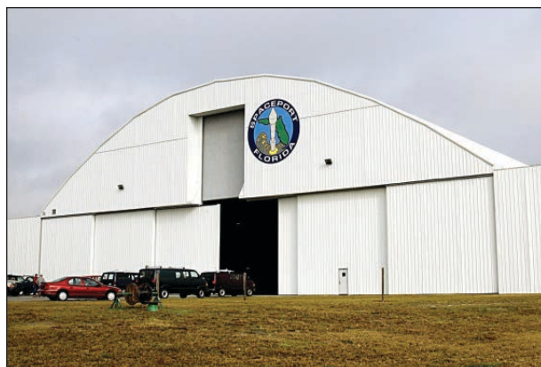
Columbia Reconstruction Hangar at the NASA Kennedy Space Center, Florida.
