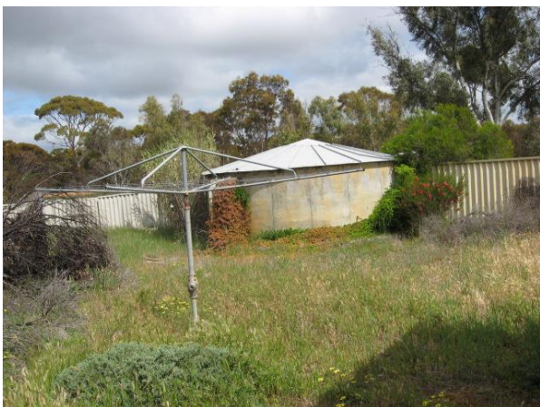
House 1; Rear yard, fibrous asbestos fence, clothes line and water tank.
