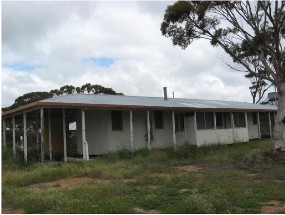
Building 8; Front view
