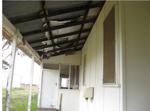
Building 8, front verandah
