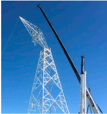
Chamouchouane–Bout-de-l'Île project: installation of the first tower in section 3, at Réservoir Taureau in Saint-Zénon (Mauricie region). Completion is slated for 2018.
