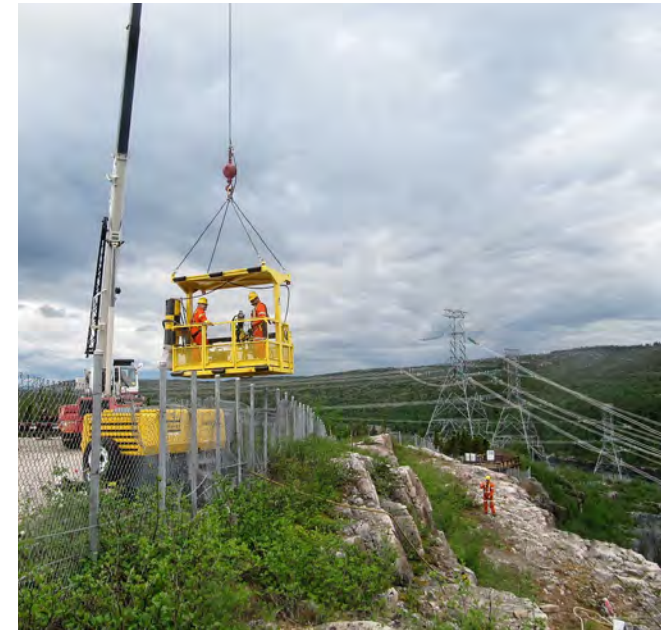
An aerial work basket with a built-in multidirectional drill, designed by the Direction – Production team in Saguenay–Lac-Saint-Jean, will be a finalist at the CNESST national OHS awards gala.
