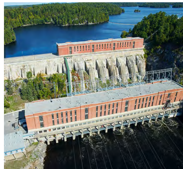
Paugan generating station (226 MW) on the Rivière Gatineau, not far from the town of Low in the Outaouais region, has been in operation since 1928—that’s 90 years! It stands as a testament to the care we take to ensure the long-term operability of our generating facilities.
