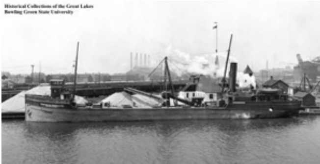
The Hennepin , after its conversion to a self-unloader.
