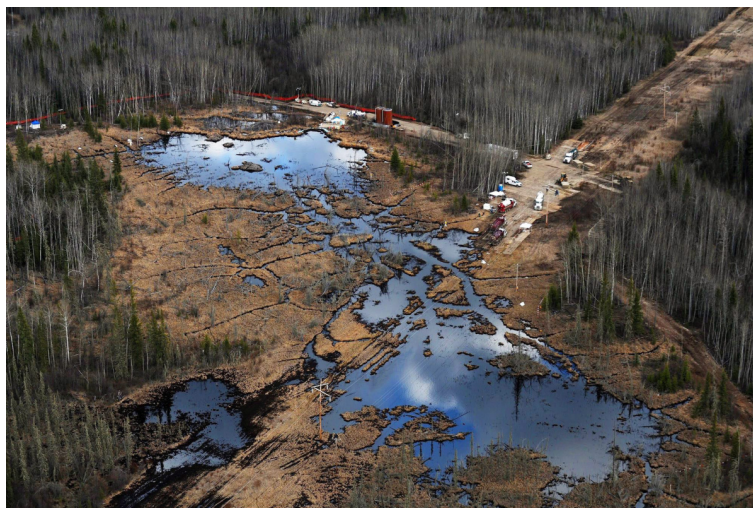
Figure 3.5: Pipeline spill northeast of Peace River, Alberta, on May 4th 2011. Source: Global News
