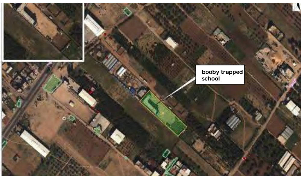
Aerial photograph of the booby trapped school (marked with arrow) in Zeitoun of Gaza City.
