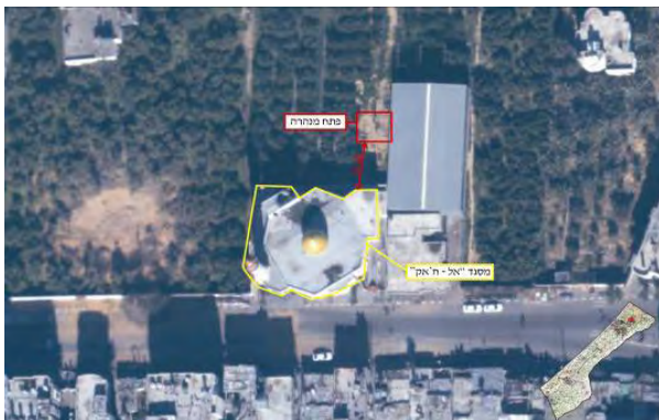
Tunnel opening near a mosque in Jabaliya, identified during Operation Cast Lead.
