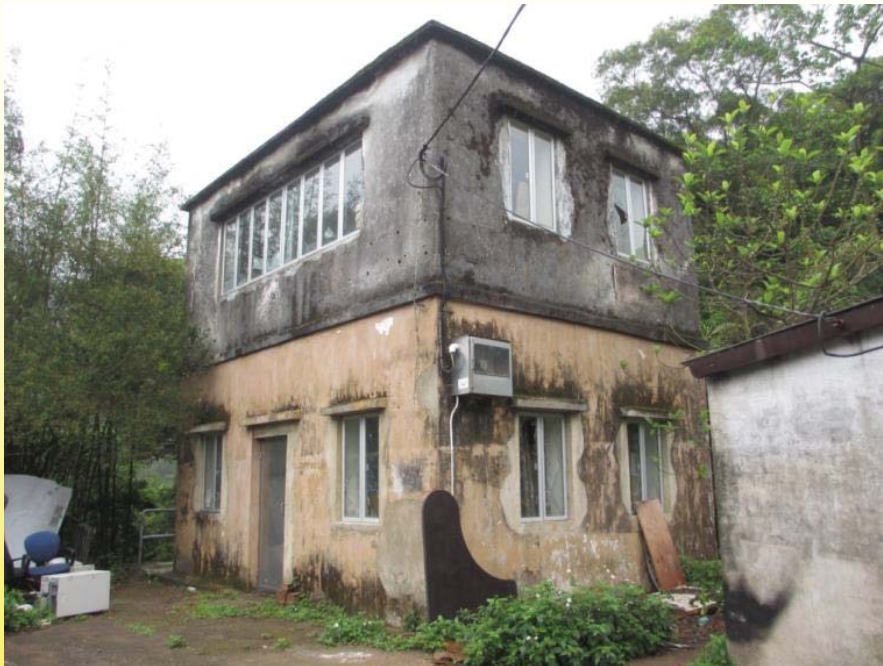
技工宿舍 Technical Staff Dormitory
