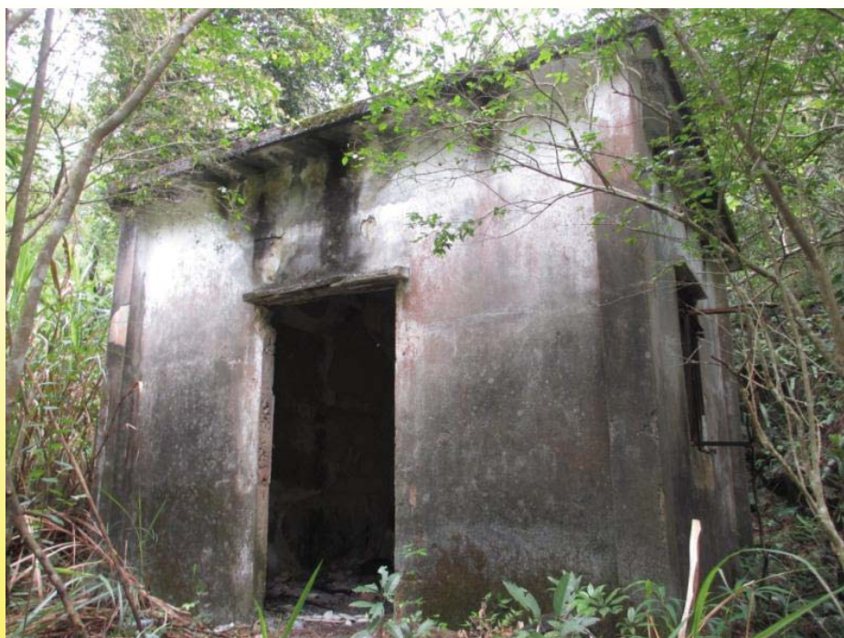
風機房 Compressed Air Generator House
